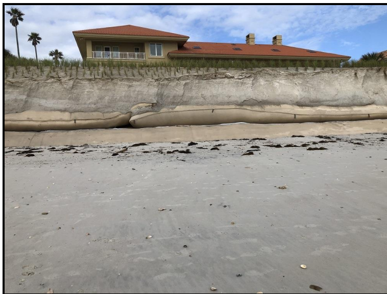
Image 5. Geotubes installed at 1085 Ponte Vedra Boulevard
