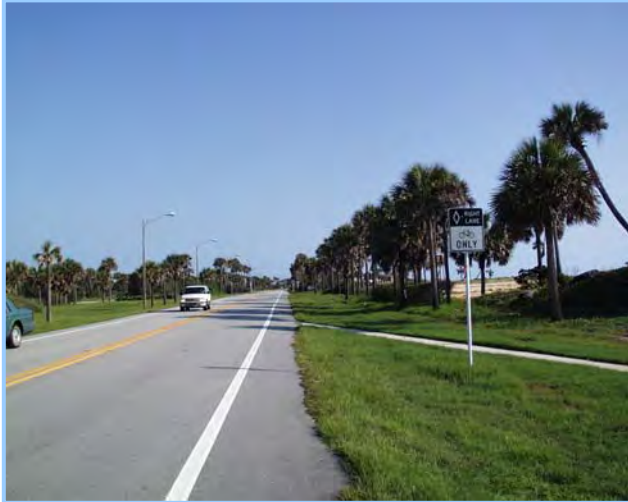
S.R. A1A, Looking North
