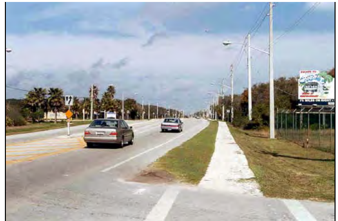
Overhead utilities along SR A1A
