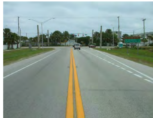
Existing, SR A1A looking east toward Vilano Beach Town Center
