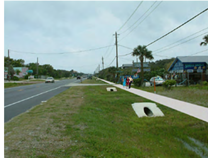
After sidewalk installation
