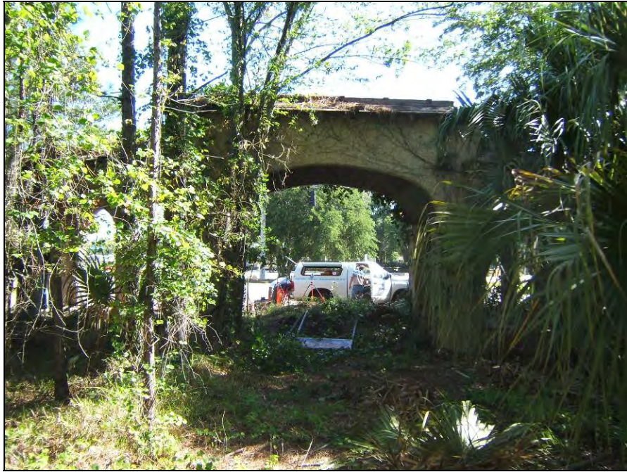
View of Arch Looking Northeast from Campus
