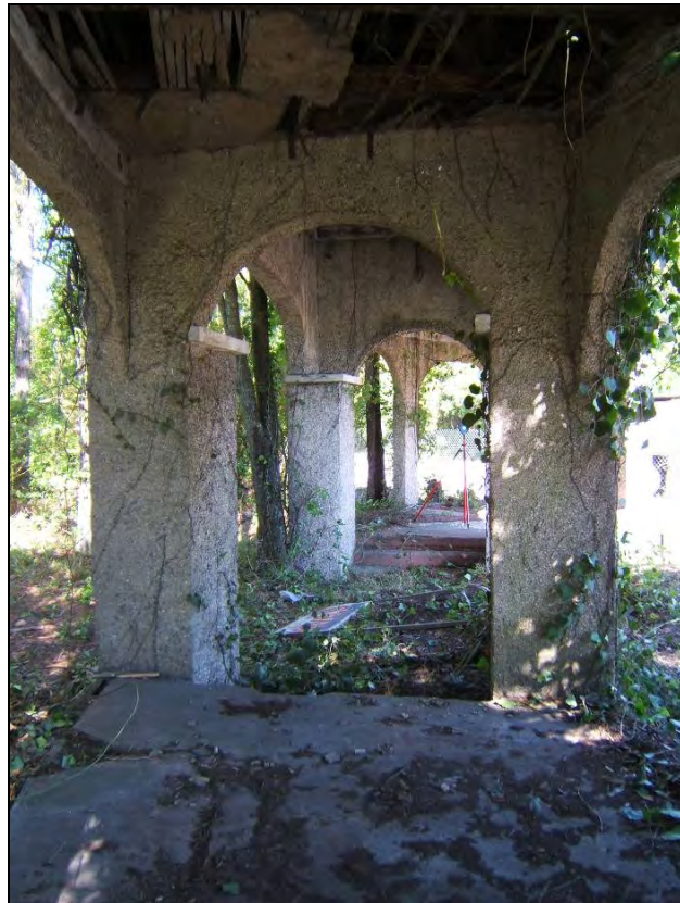
View of Arch from inside Looking Northwest
