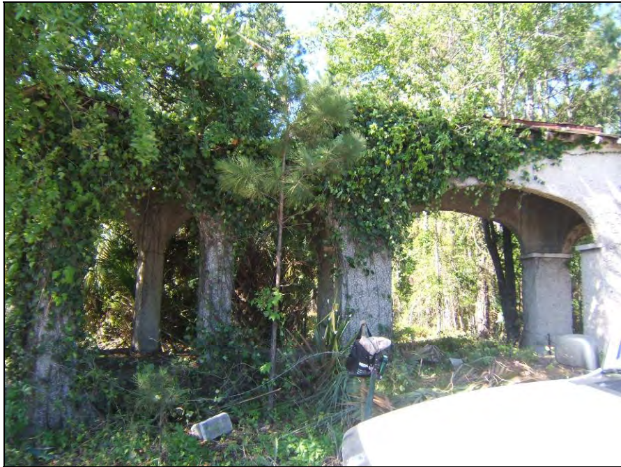
View of Arch Looking Southwest
