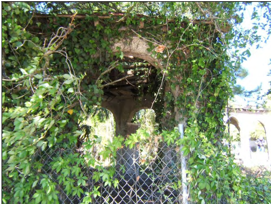
View of Arch Looking West
