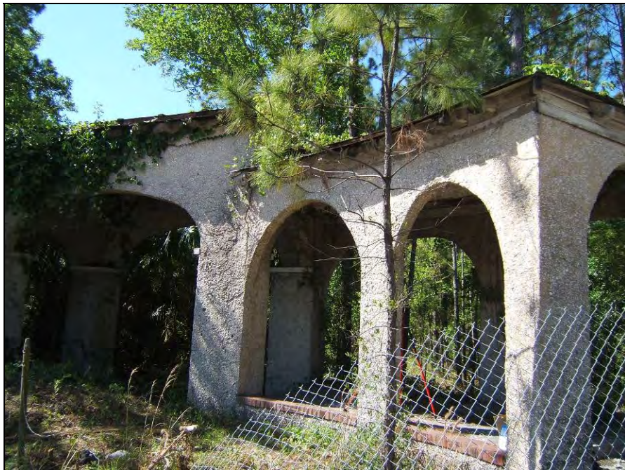
View of Arch Looking South
