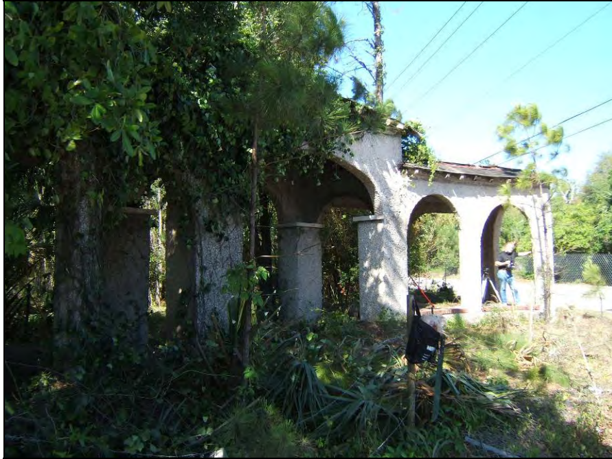
View of Arch Looking West-Northwest
