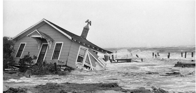
Jacksonville Beach - 1964 Hurricane "Dora"
