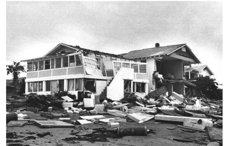
Jacksonville Beach - 1964 Hurricane "Dora"
