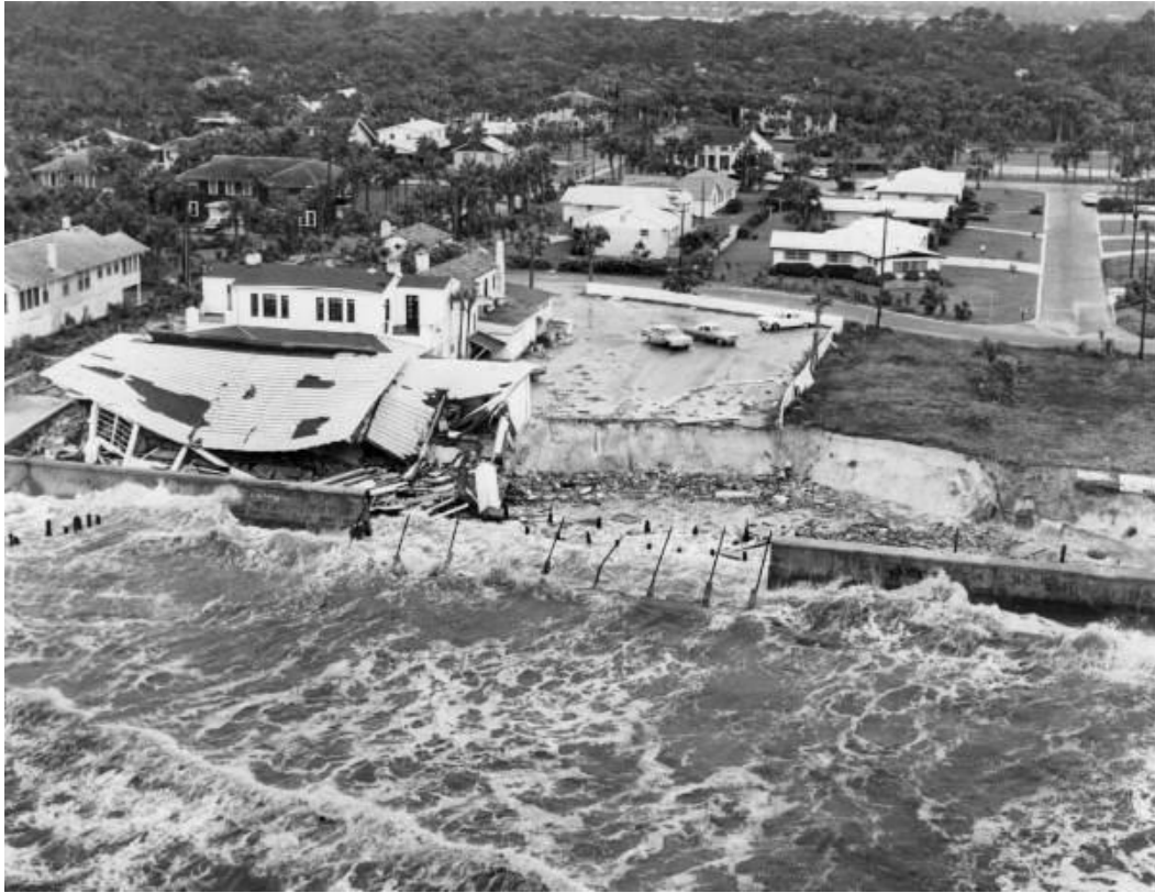
Jacksonville Beach - 1964 Hurricane "Dora"
