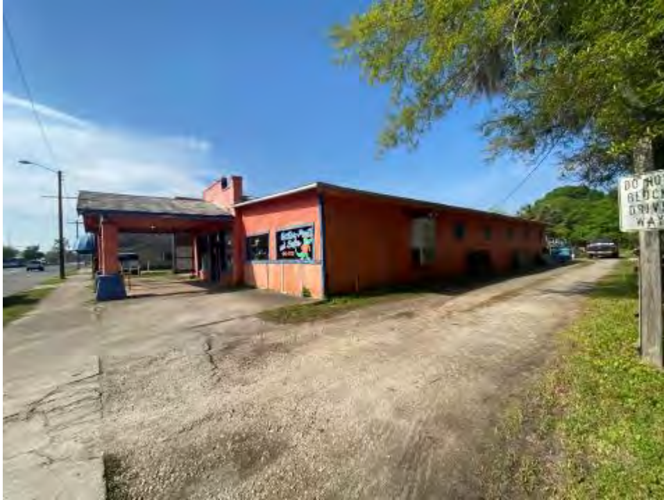
Figure 1131. Photograph of SJ07953 – 1 facing southwest.
