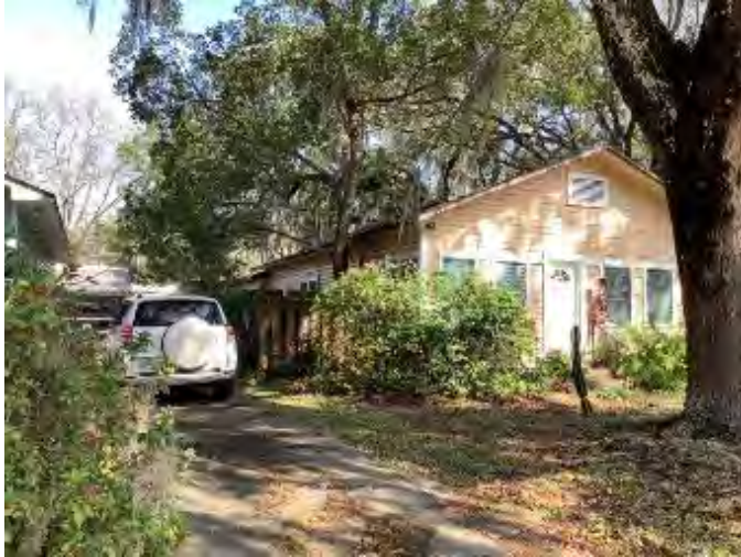
Figure 127. Photograph of SJ02672 – 3 facing east.
