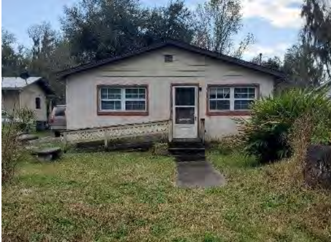
Figure 565. Photograph of SJ07786 – 1 facing south.
