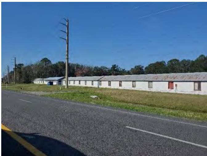
Figure 248. Photograph of SJ03546 – Building A SJ035408, 2 facing southwest.
