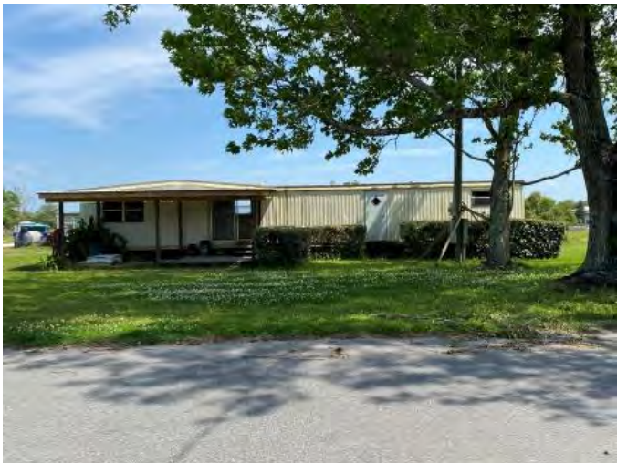
Figure 1206. Photograph of SJ07973 – 2 facing east.
