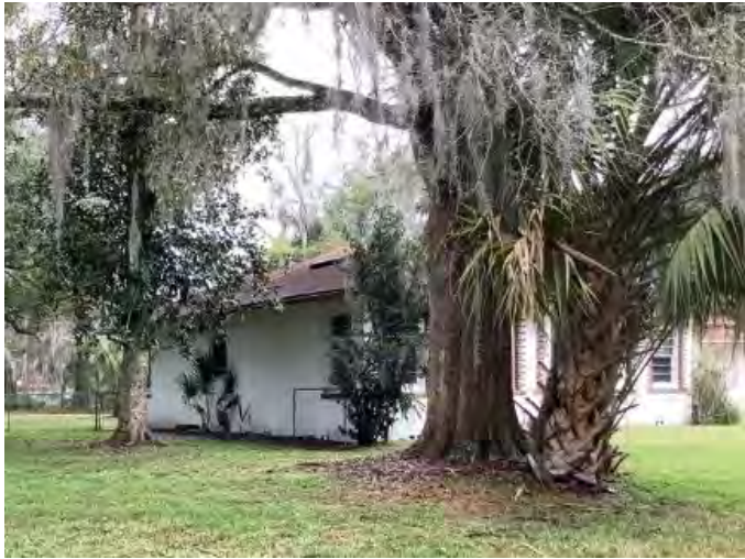
Figure 581. Photograph of SJ07791 – 2 facing east.
