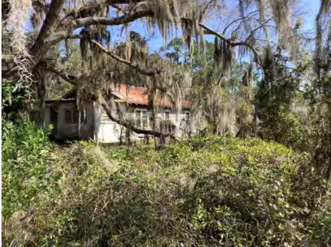
Figure 1019. Photograph of SJ07923 – 1 facing east.
