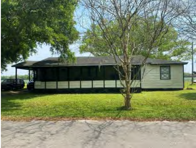
Figure 1235. Photograph of SJ07980 – 3 facing east.
