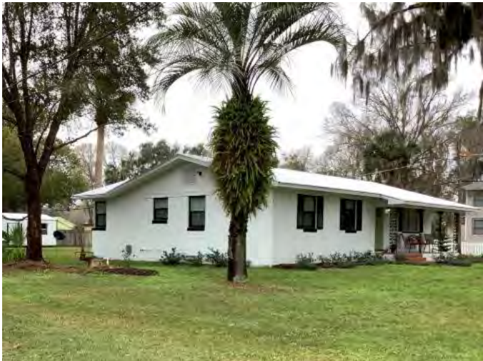
Figure 493. Photograph of SJ07766 – 2 facing west.
