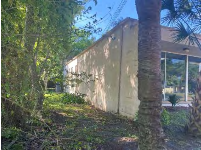
Figure 1072. Photograph of SJ07937 – 1 facing southwest.
