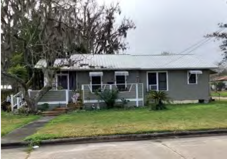
Figure 637. Photograph of SJ07806 – 2 facing south.
