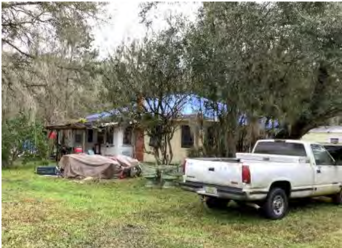
Figure 686. Photograph of SJ078189- 2 facing east.
