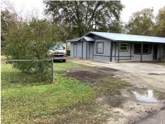
Figure 727. Photograph of SJ07831 – 3 facing east.
