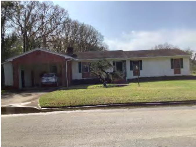
Figure 383. Photograph of SJ07733 – 1 facing south.
