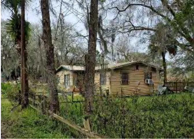
Figure 594. Photograph of SJ07795– 1 facing northwest.
