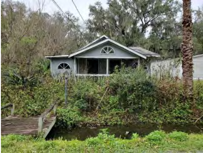
Figure 863. Photograph of SJ07872 – 1 facing west.
