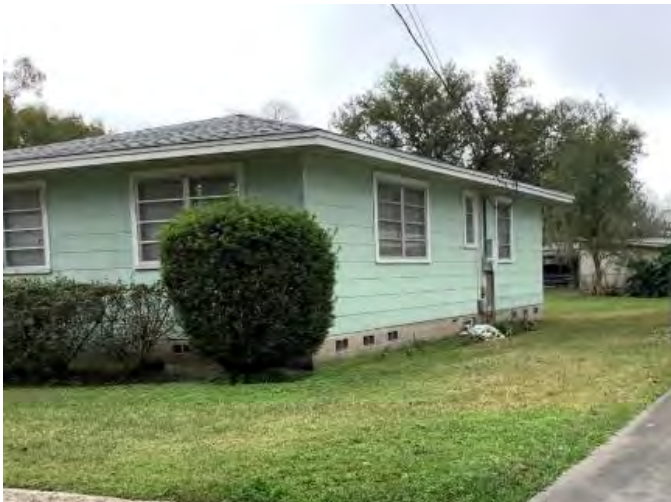
Figure 588. Photograph of SJ07793 – 2 facing east.
