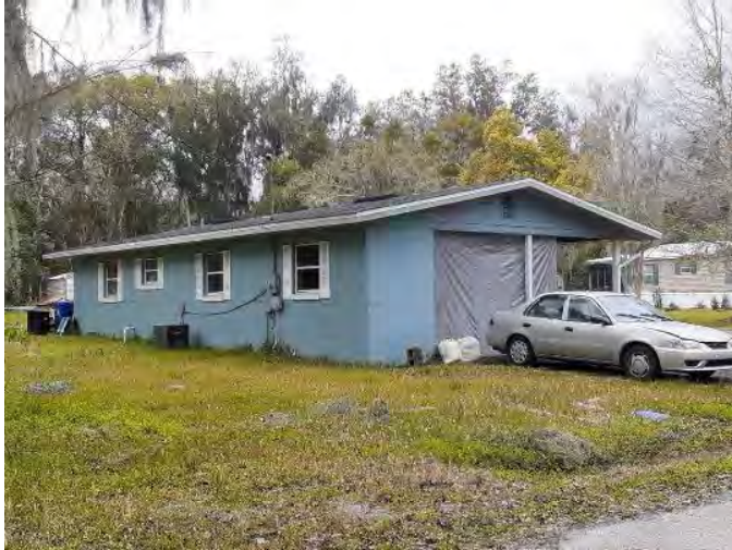
Figure 769. Photograph of SJ07844 – 1 facing west.
