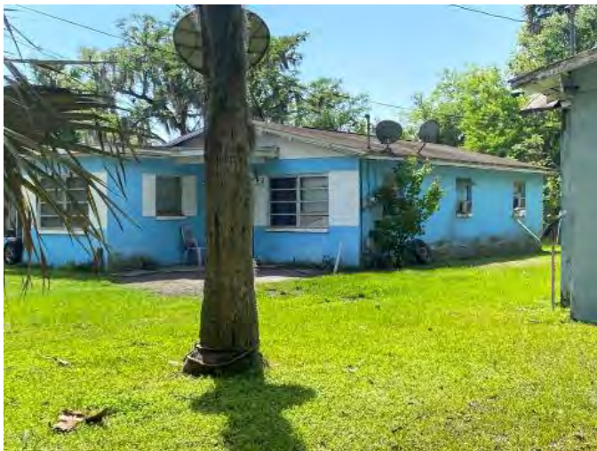
Figure 1118. Photograph of SJ07949 – 2 facing southwest.
