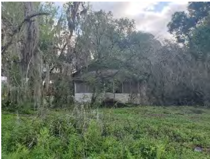
Figure 979. Photograph of SJ07910 – 1 facing east.
