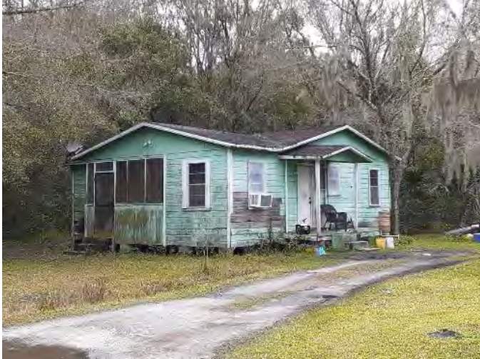
Figure 802. Photograph of SJ07854 – 1 facing southwest.
