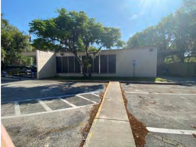
Figure 1074. Photograph of SJ07937 – 3 facing east.
