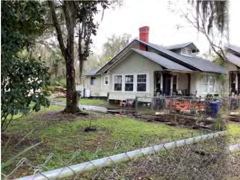
Figure 174. Photograph of SJ02685- 1 facing west.
