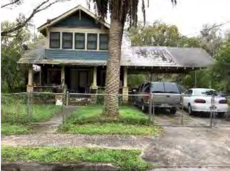
Figure 177. Photograph of SJ02686- 1 facing south.
