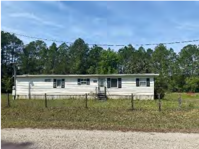
Figure 709. Photograph of SJ07827 – 2 facing west.
