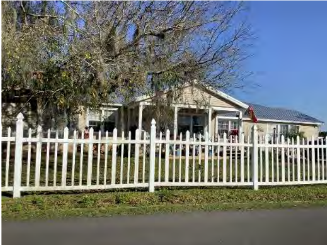
Figure 972. Photograph of SJ07908 – 2 facing east.
