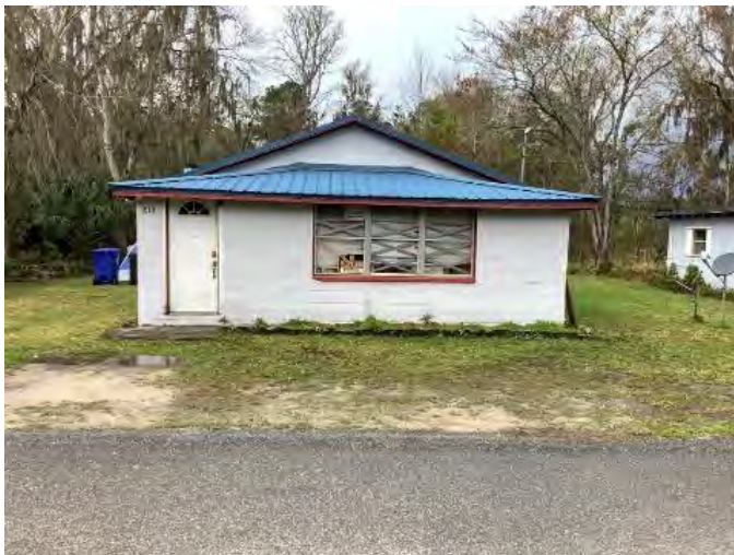
Figure 959. Photograph of SJ07904 – 2 facing west.
