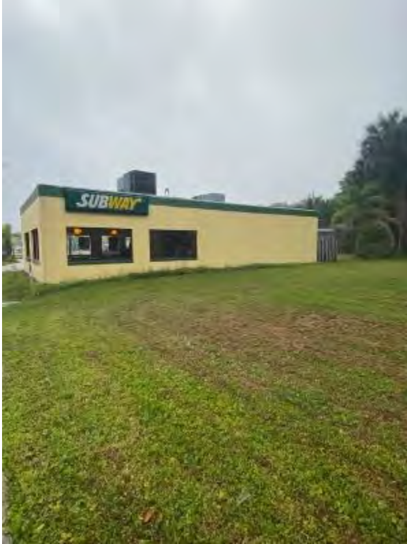
Figure 1231. Photograph of SJ07979 – 3 facing east.
