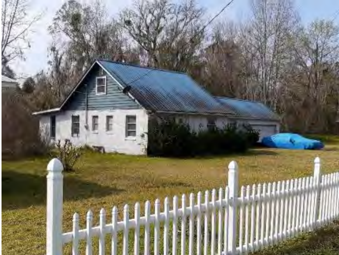
Figure 509. Photograph of SJ07770 – 1 facing southwest.
