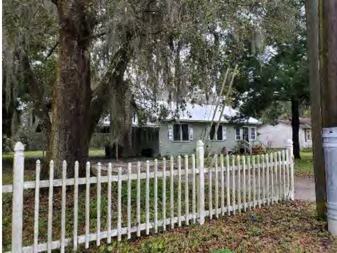
Figure 795. Photograph of SJ07851 – 3 facing southwest.
