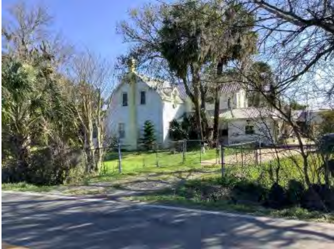
Figure 231. Photograph of SJ02880- 1 facing south.
