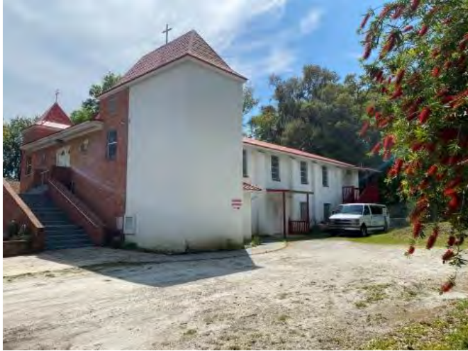
Figure 1129. Photograph of SJ07952 – 3 facing southwest.
