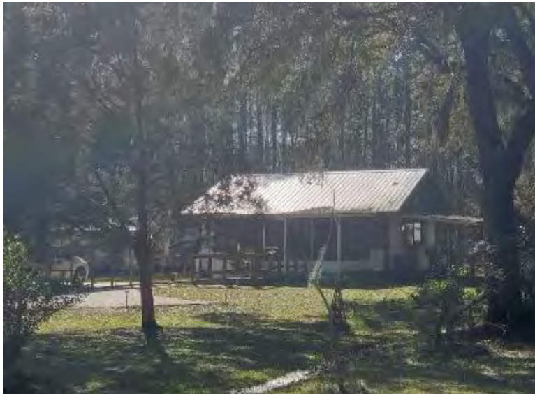
Figure 652. Photograph of SJ07810– 1 facing south.
