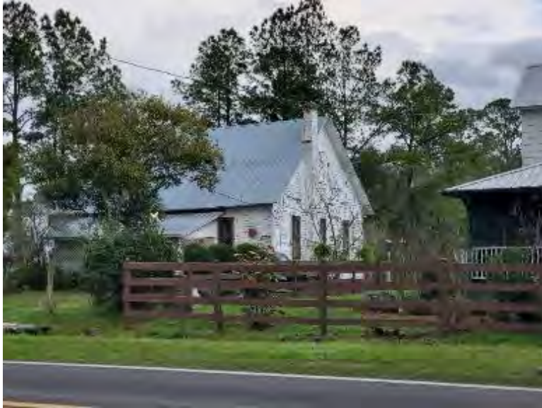
Figure 38. Photograph of SJ02587 – 3 facing east.
