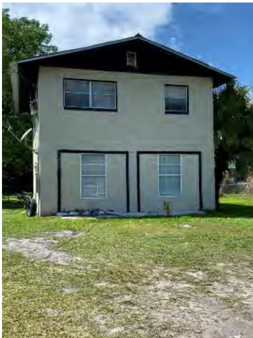
Figure 1142. Photograph of SJ07955 – 2 facing west.
