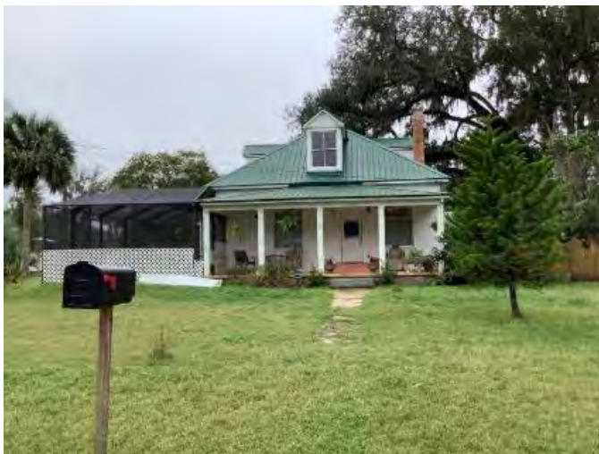
Figure 117. Photograph of SJ02668 – 1 facing south.
