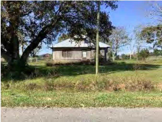
Figure 225. Photograph of SJ02873 – 2 facing west.
