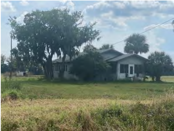
Figure 1196. Photograph of SJ07970 – 3 facing southwest.
