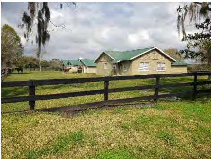
Figure 916. Photograph of SJ07890 – 2 facing east.
