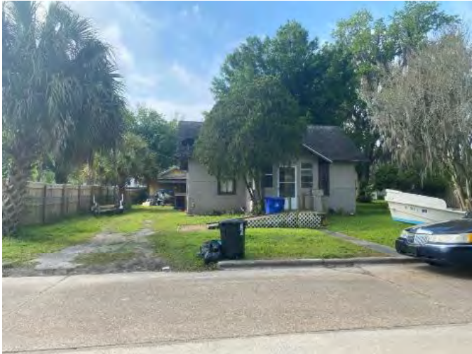
Figure 1091. Photograph of SJ07942 – 2 facing south.
