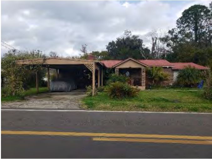
Figure 574. Photograph of SJ07789— 1 northeast
