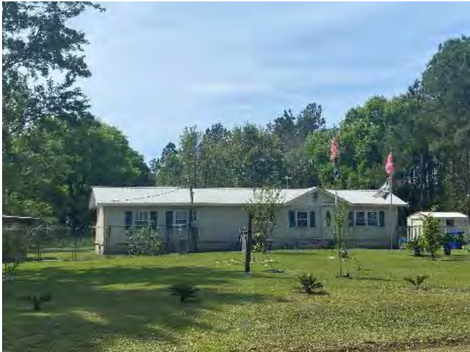
Figure 739. Photograph of SJ07835 – 1 facing south.
