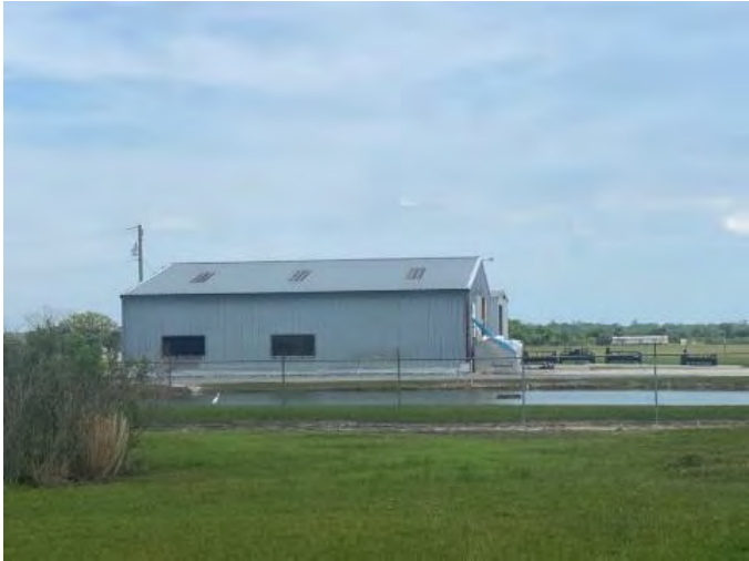
Figure 1201. Photograph of SJ07972 – 1 facing east.
