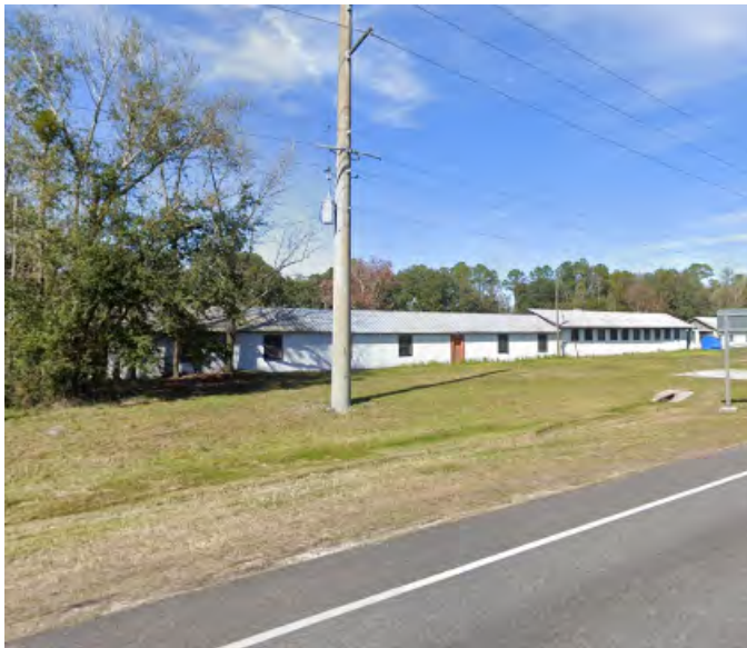
Figure 250. Photograph of SJ03546 – Building B SJ035409, 2 facing northwest.
