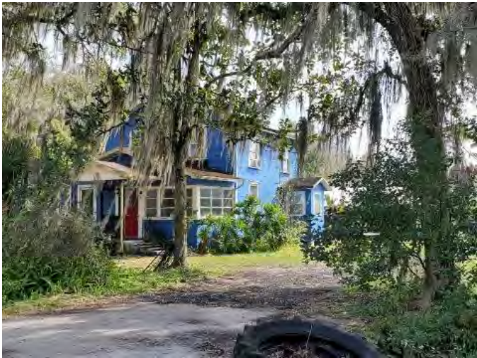
Figure 320. Photograph of SJ04244- 1 facing east.
