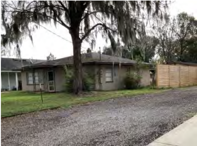
Figure 614. Photograph of SJ07800 – 3 facing east.
