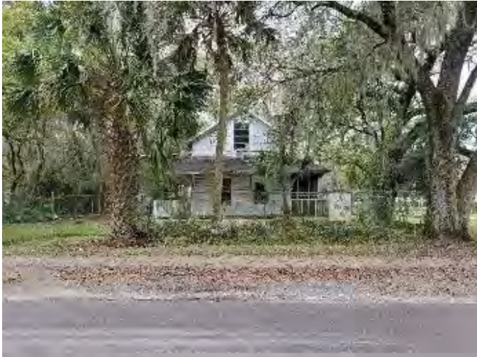
Figure 79. Photograph of SJ02651 – 2 facing west.
