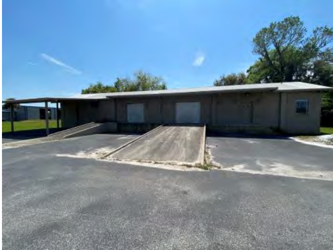
Figure 1222. Photograph of SJ07977 – 2 facing south.
