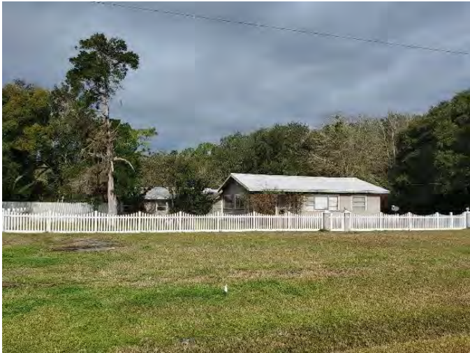
Figure 787. Photograph of SJ07849 – 3 facing northwest.
