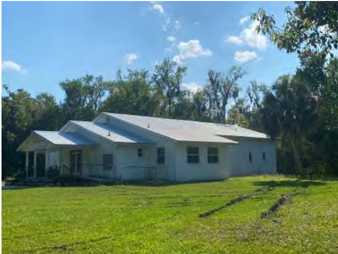
Figure 1166. Photograph of SJ07961 – 3 facing southwest.
