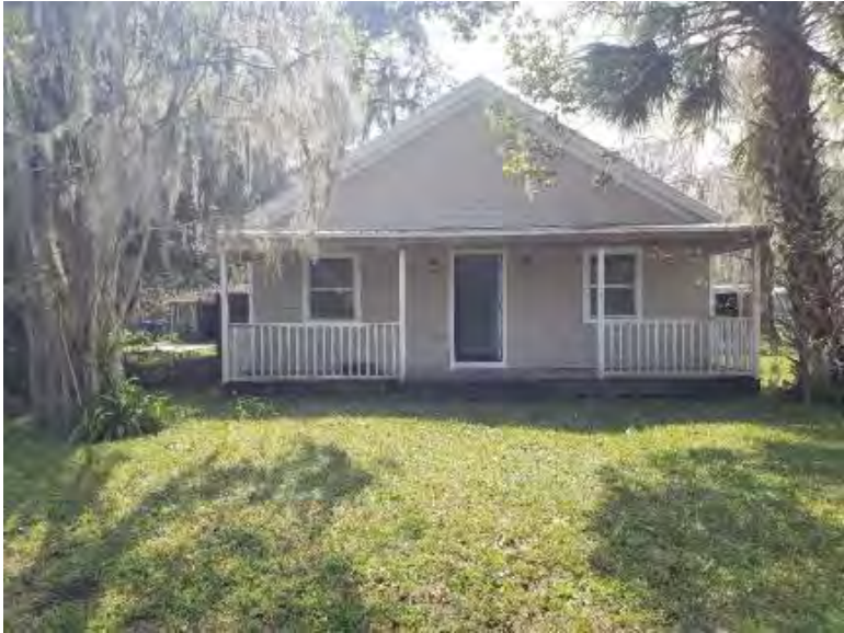
Figure 644. Photograph of SJ07808– 1 facing south.
