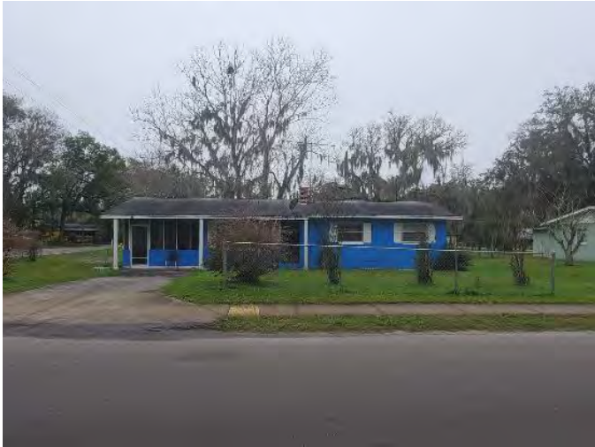
Figure 821. Photograph of SJ07859 – 2 facing east.
