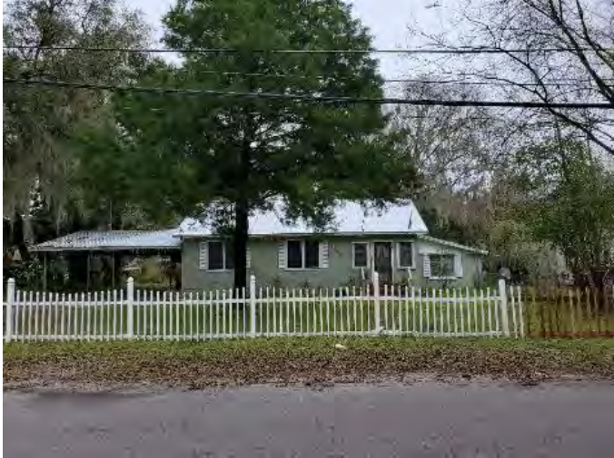
Figure 794. Photograph of SJ07851 – 2 facing west.
