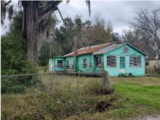
Figure 844. Photograph of SJ07865 – 3 facing east.
