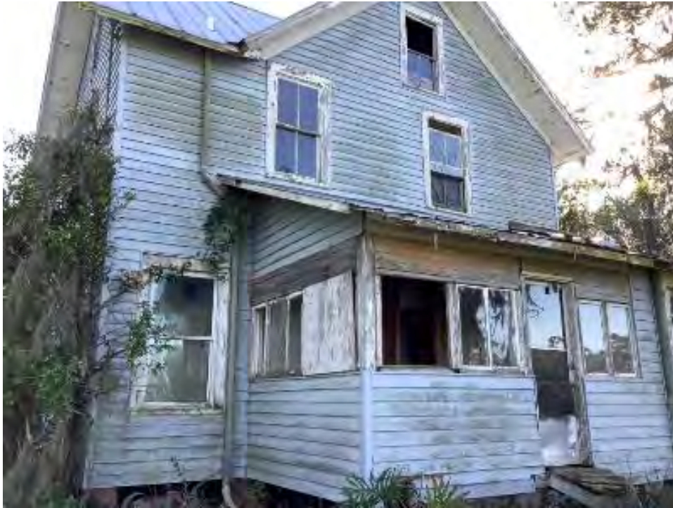
Figure 13. Photograph of SJ02572 – 3 facing southwest.
