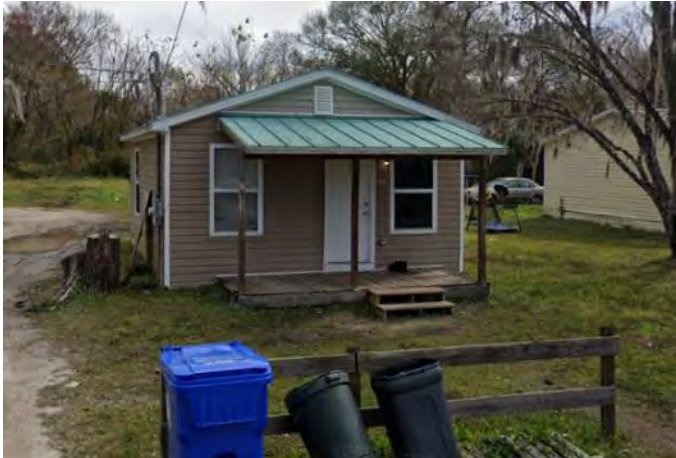
Figure 1173. Photograph of SJ07963 – 2 facing east.
