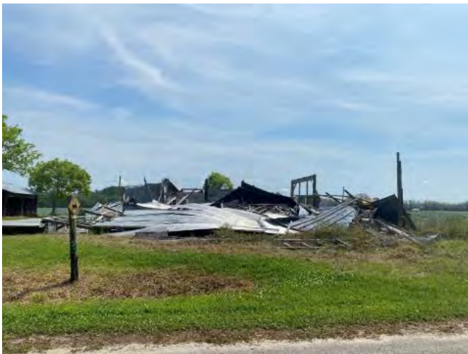
Figure 1236. Photograph of SJ07980 outbuilding– 4 facing southeast.
