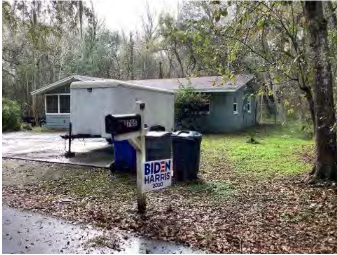
Figure 926. Photograph of SJ07893 – 1 facing west.
