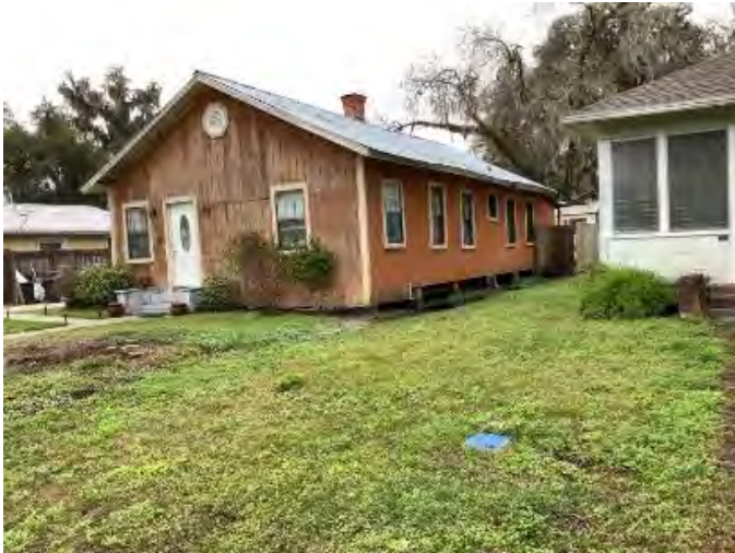
Figure 186. Photograph of SJ02688 – 3 facing west.
