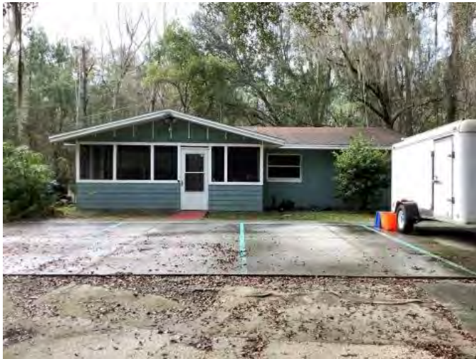
Figure 927. Photograph of SJ07893 – 2 facing southwest.
