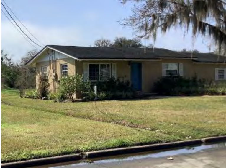
Figure 438. Photograph of SJ07749 – 3 facing southwest.
