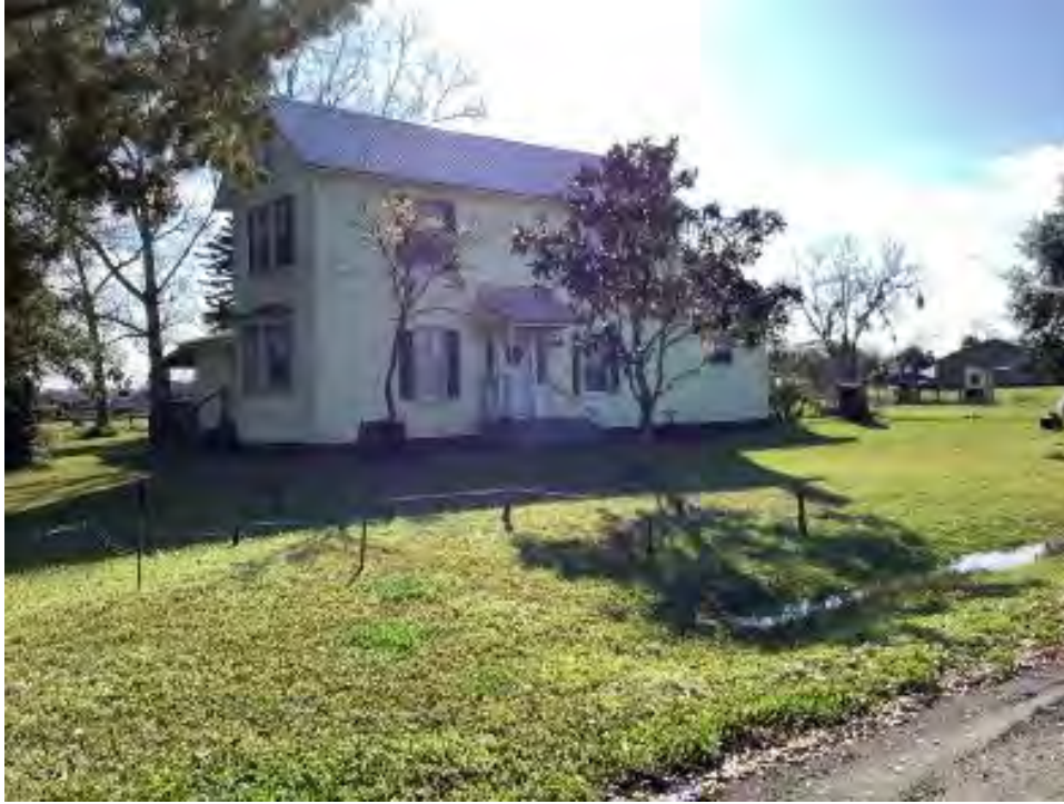
Figure 19. Photograph of SJ02578 – 1 facing east.
