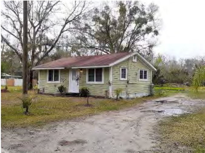
Figure 847. Photograph of SJ07866 – 2 facing southwest.
