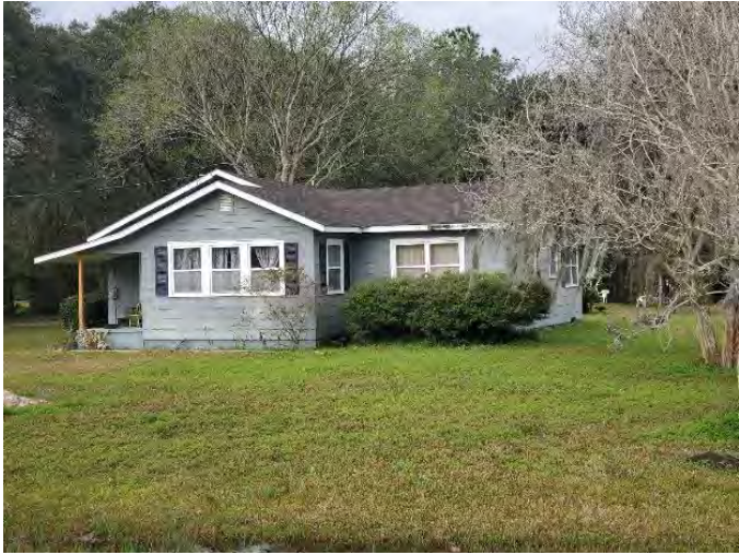
Figure 758. Photograph of SJ07841 – 1 facing southwest.
