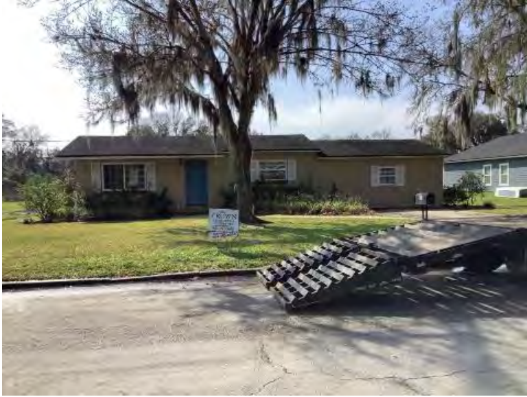
Figure 436. Photograph of SJ07749 – 1 facing south.
