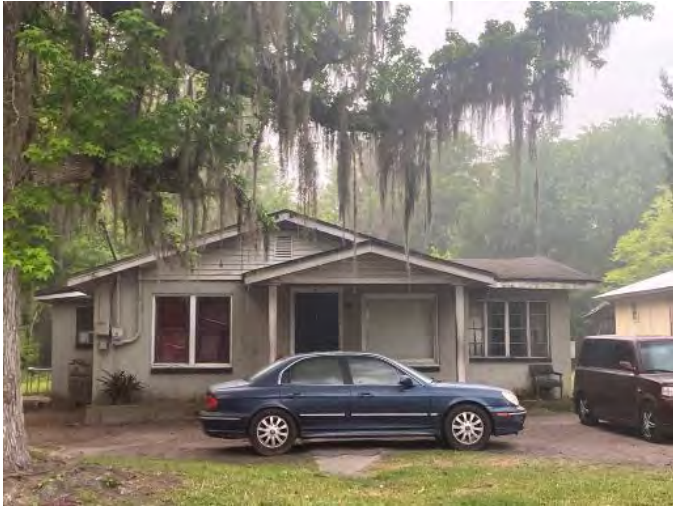
Figure 1077. Photograph of SJ07938 – 2 facing south.
