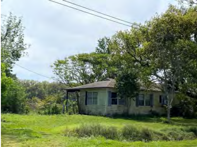
Figure 1159. Photograph of SJ07960 – 1 facing southwest.
