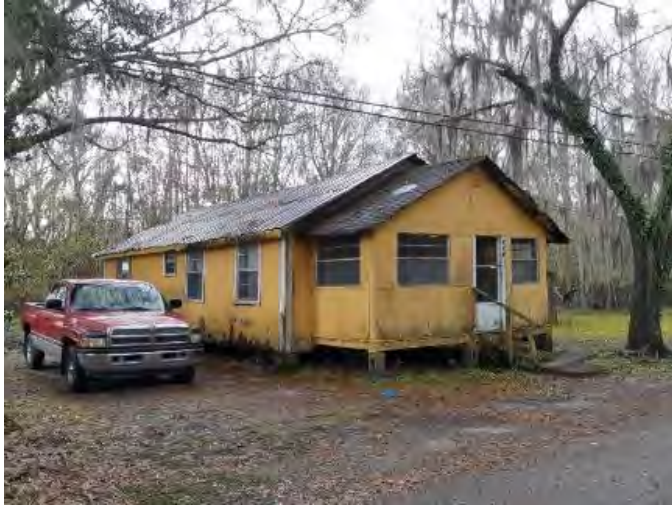
Figure 600. Photograph of SJ07796 – 3 facing southwest.
