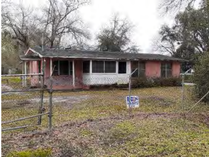
Figure 1004. Photograph of SJ07917 – 1 facing southwest.
