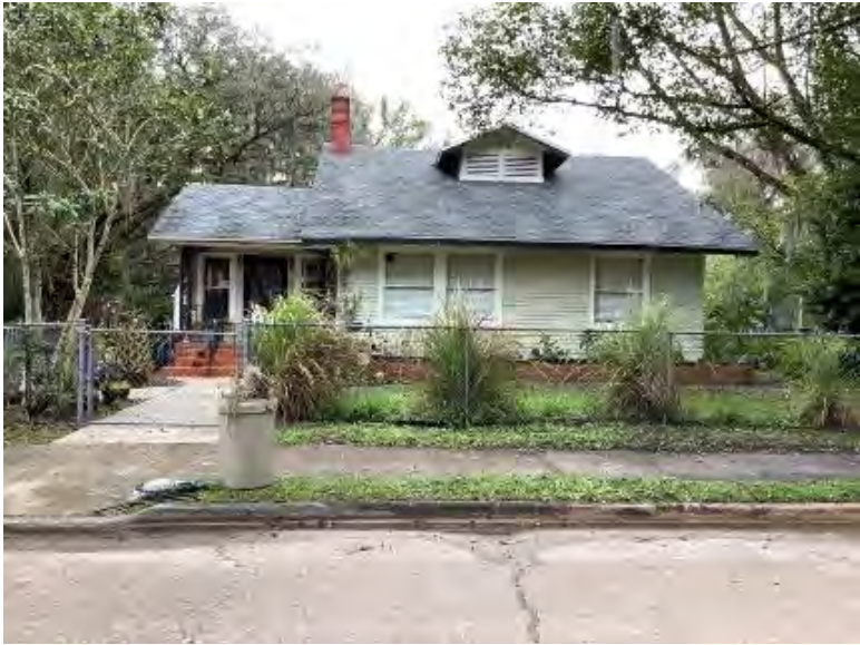
Figure 175. Photograph of SJ02685 – 2 facing south.
