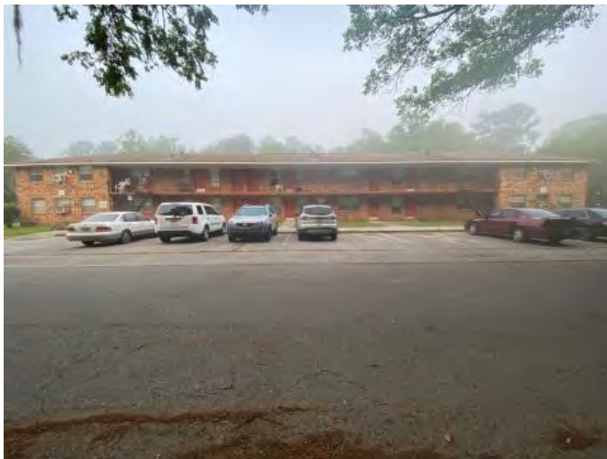
Figure 1184. Photograph of SJ07966 – 2 facing west.
