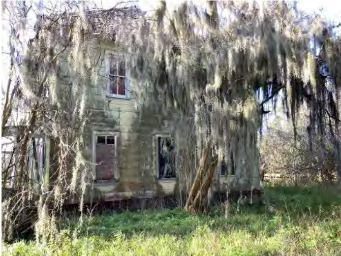
Figure 331. Photograph of SJ04252 – 4 facing south.
