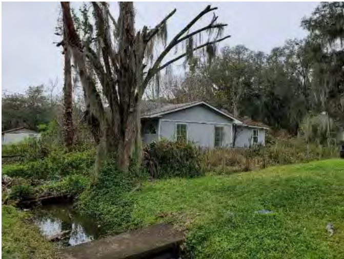
Figure 864. Photograph of SJ07872 – 2 facing southwest.
