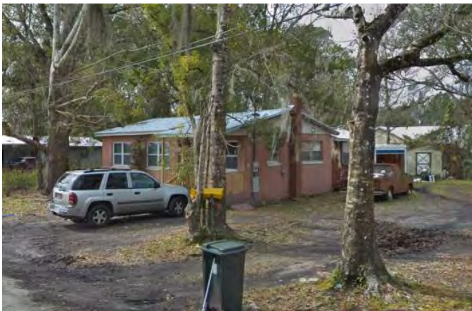
Figure 934. Photograph of SJ07895 – 2 facing southwest.
