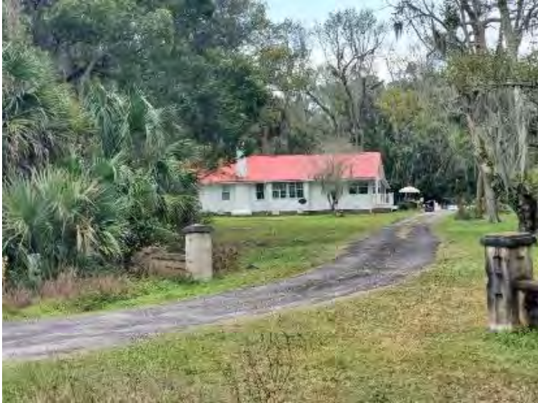
Figure 42. Photograph of SJ02591 – 1 facing south.
