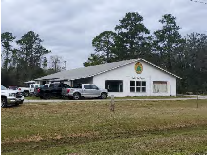
Figure 729. Photograph of SJ07832 – 1 facing northwest.
