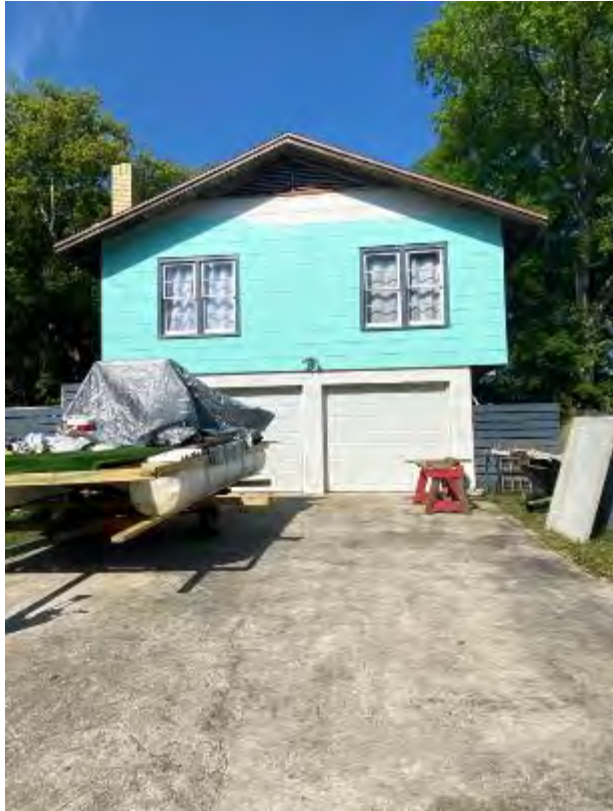
Figure 1057. Photograph of SJ07933 – 2 facing west.
