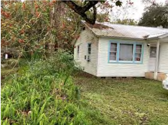
Figure 659. Photograph of SJ07812 – 2 facing west.
