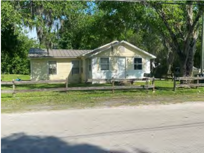
Figure 1169. Photograph of SJ07962 – 2 facing east.
