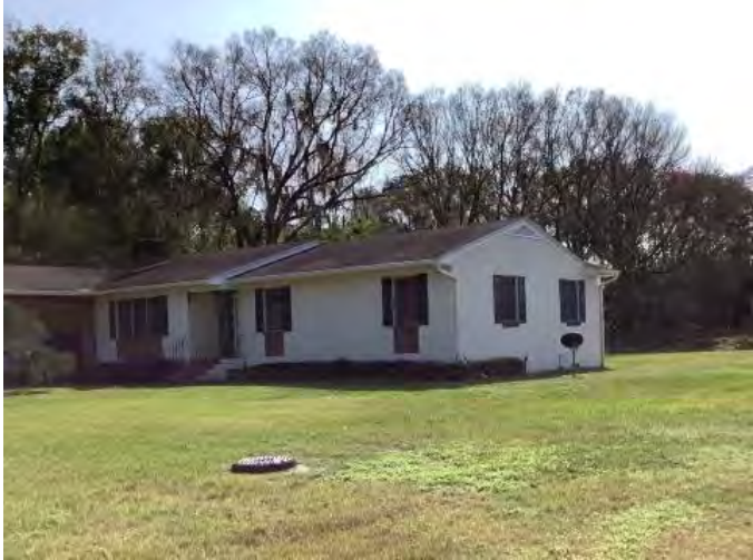
Figure 384. Photograph of SJ07733– 2 facing east.
