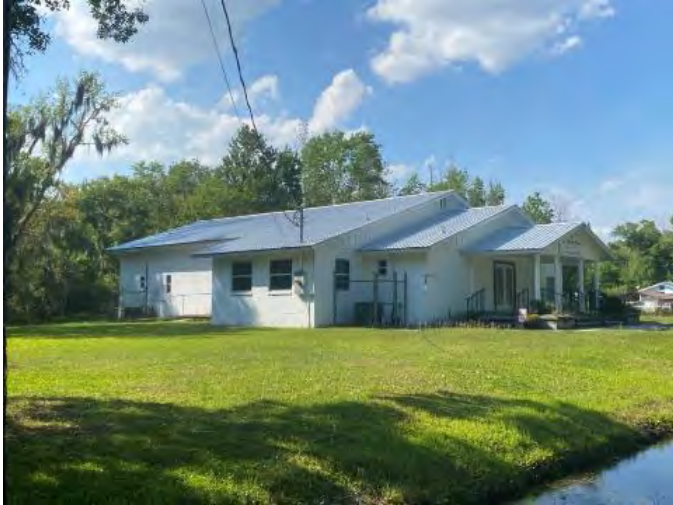
Figure 1164. Photograph of SJ07961 – 1 facing northwest.
