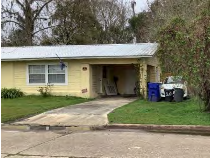
Figure 370. Photograph of SJ07729 – 3 facing west.
