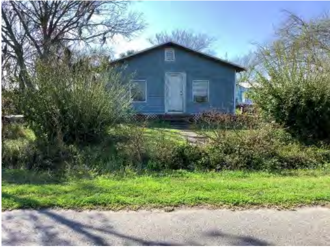
Figure 824. Photograph of SJ07860 – 1 facing east.
