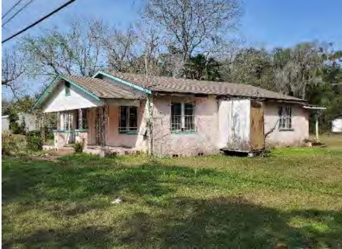
Figure 592. Photograph of SJ07794 – 3 facing northwest.
