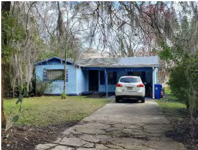
Figure 797. Photograph of SJ07852 – 1 facing east.
