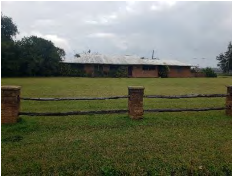
Figure 886. Photograph of SJ07880 – 1 facing east.
