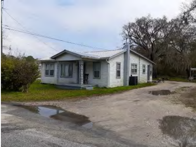
Figure 941. Photograph of SJ07898 – 1 facing east.
