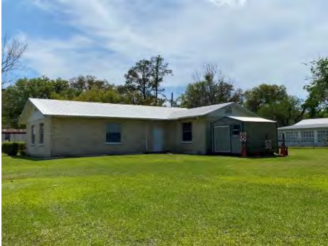
Figure 1120. Photograph of SJ07950 – 1 facing southwest.
