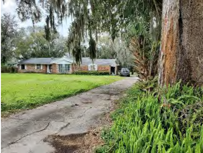
Figure 896. Photograph of SJ07884 – 1 facing south.
