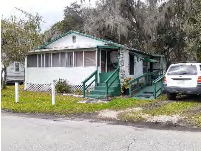
Figure 434. Photograph of SJ07748 – 3 facing northwest.
