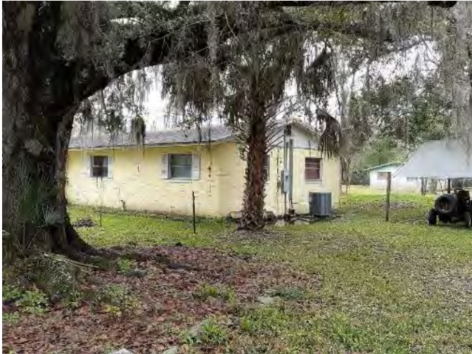
Figure 829. Photograph of SJ07861 – 2 facing southwest.
