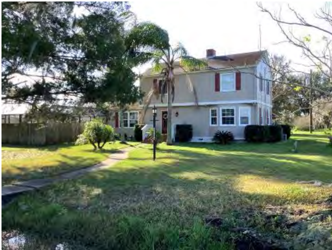
Figure 875. Photograph of SJ07876 – 2 facing south.
