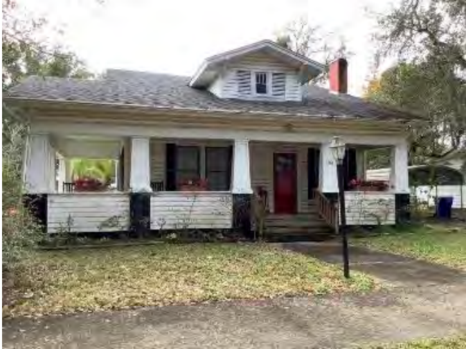
Figure 142. Photograph of SJ02677– 1 facing west.
