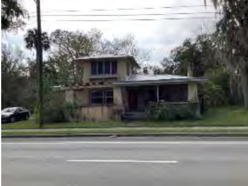
Figure 64. Photograph of SJ02600 – 3 facing south.
