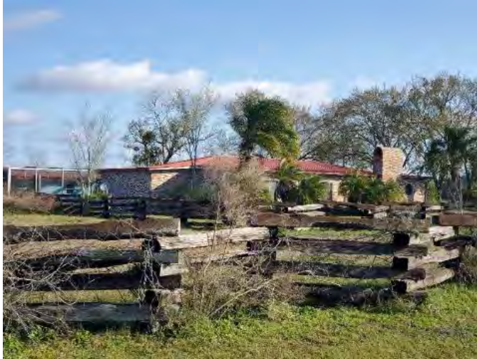
Figure 1011. Photograph of SJ07919 – 3 facing northwest.
