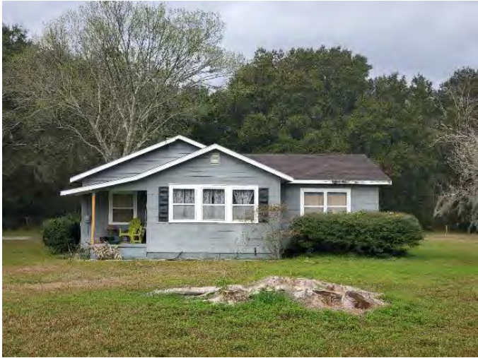
Figure 759. Photograph of SJ07841 – 2 facing west.
