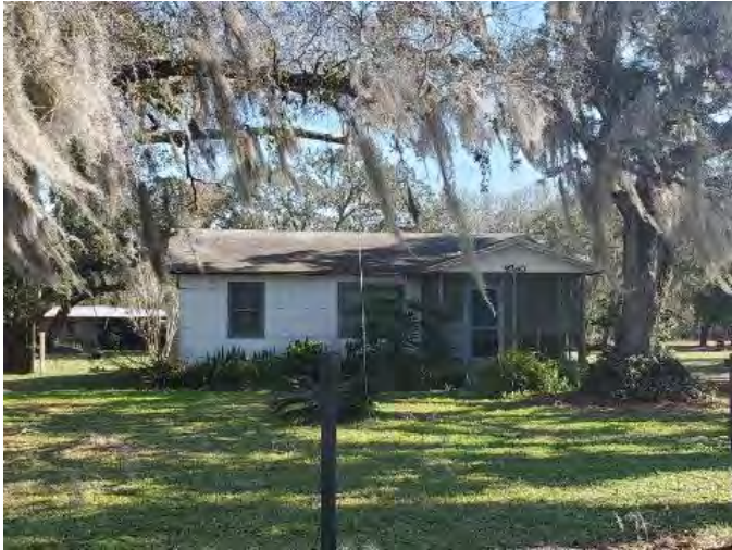
Figure 1038. Photograph of SJ07928 – 2 facing south.
