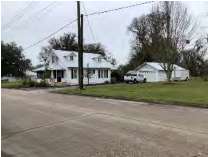
Figure 95. Photograph of SJ02658 – 3 facing east.
