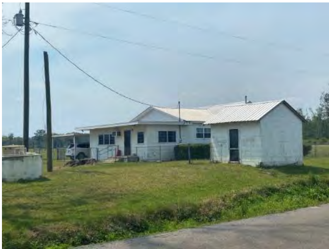
Figure 1245. Photograph of SJ07983 – 2 facing southwest.
