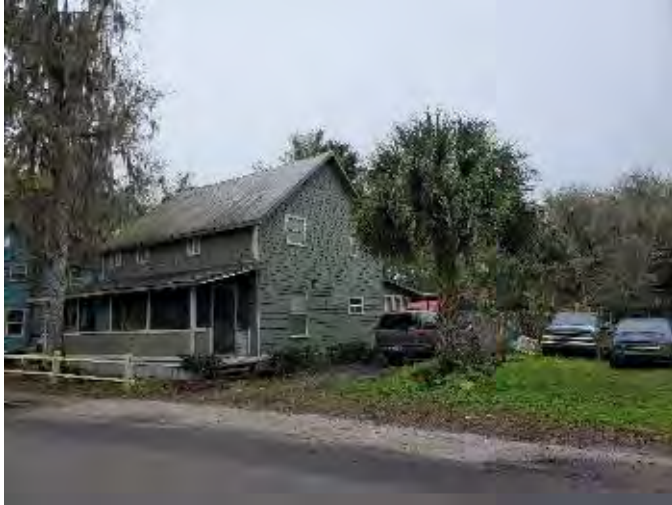
Figure 88. Photograph of SJ02653 – 3 facing southwest.
