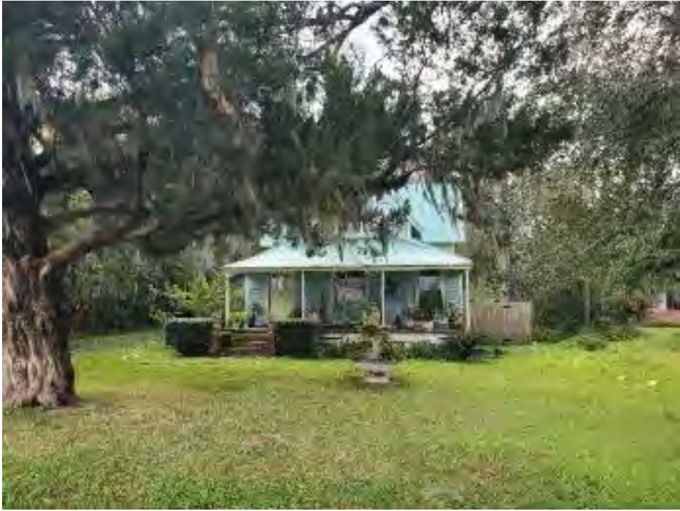
Figure 53. Photograph of SJ02595 – 2 facing west.
