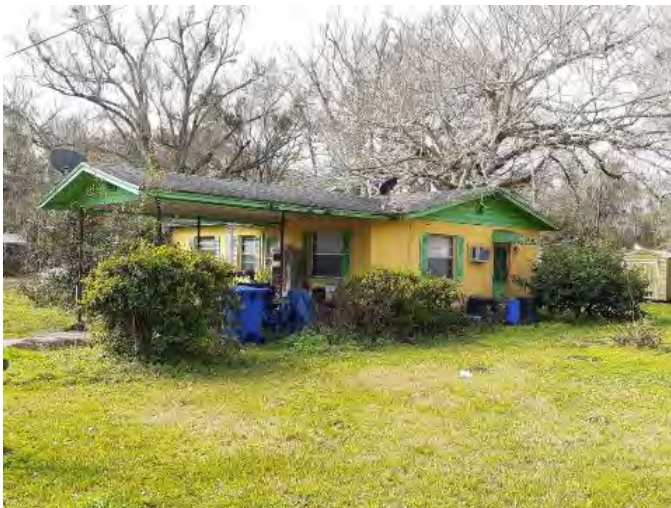
Figure 939. Photograph of SJ07897 – 2 facing southwest.
