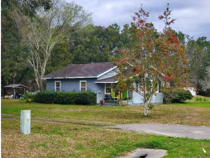
Figure 760. Photograph of SJ07841 – 3 facing northwest.
