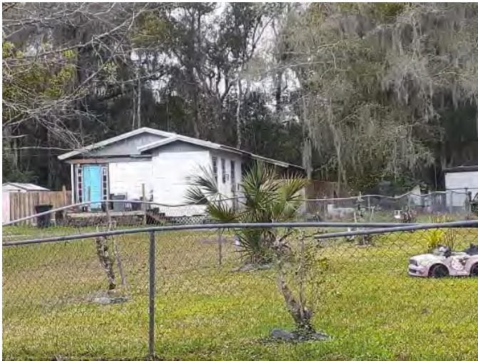
Figure 773. Photograph of SJ07845 – 2 facing southwest.
