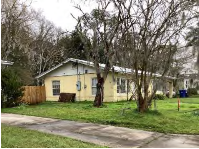
Figure 369. Photograph of SJ07729 – 2 facing east.
