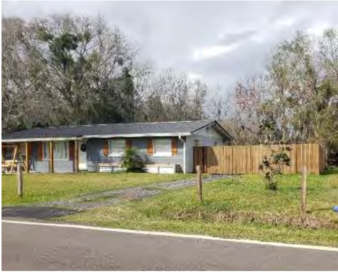
Figure 572. Photograph of SJ07788 – 2 facing northwest.
