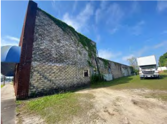
Figure 1109. Photograph of SJ07947– 1 facing southwest.
