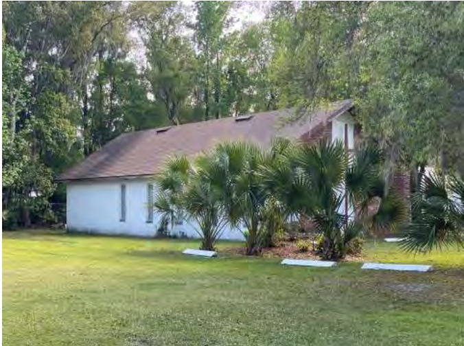
Figure 1113. Photograph of SJ07948 – 1 facing southwest.
