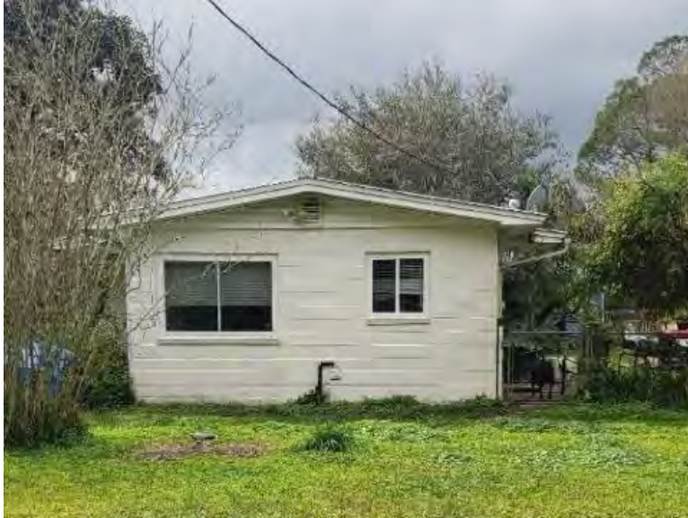
Figure 464. Photograph of SJ07757 – 3 facing southwest.
