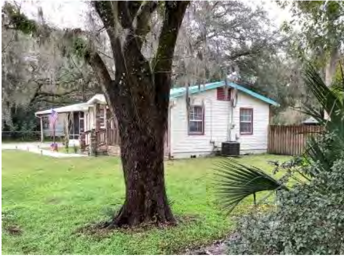
Figure 672. Photograph of SJ07815 – 3 facing east.
