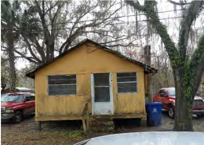
Figure 599. Photograph of SJ07796 - 2 facing south.
