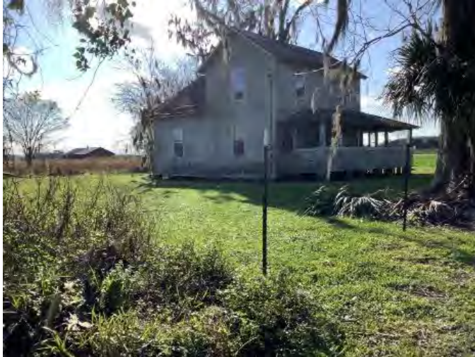
Figure 3. Photograph of SJ02567 – 3 facing south.
