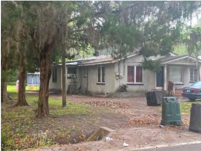
Figure 1078. Photograph of SJ07938 – 3 facing southwest.
