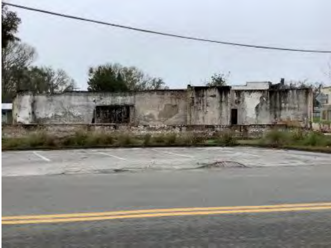
Figure 201. Photograph of SJ02701 – 3 facing south.
