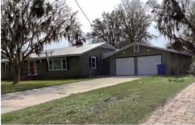
Figure 516. Photograph of SJ07772 – 1 facing east.
