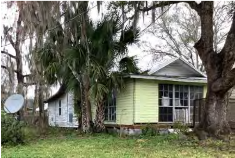
Figure 625. Photograph of SJ07803 – 2 facing east.
