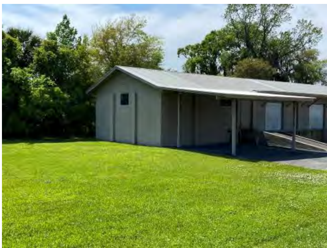
Figure 1221. Photograph of SJ07977 – 1 facing southwest.
