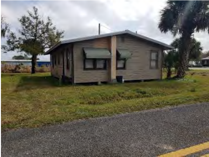
Figure 983. Photograph of SJ07911 – 2 facing east.
