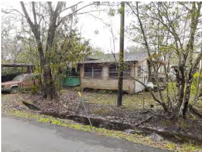
Figure 850. Photograph of SJ07867 – 2 facing southwest.
