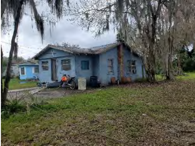
Figure 312. Photograph of SJ04236– 1 facing south.
