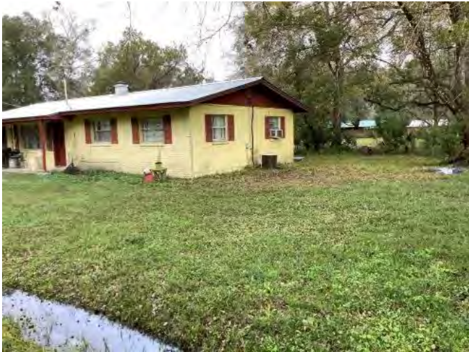
Figure 743. Photograph of SJ07836 – 2 facing west.
