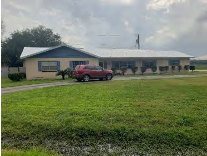
Figure 762. Photograph of SJ07842 – 1 facing east.
