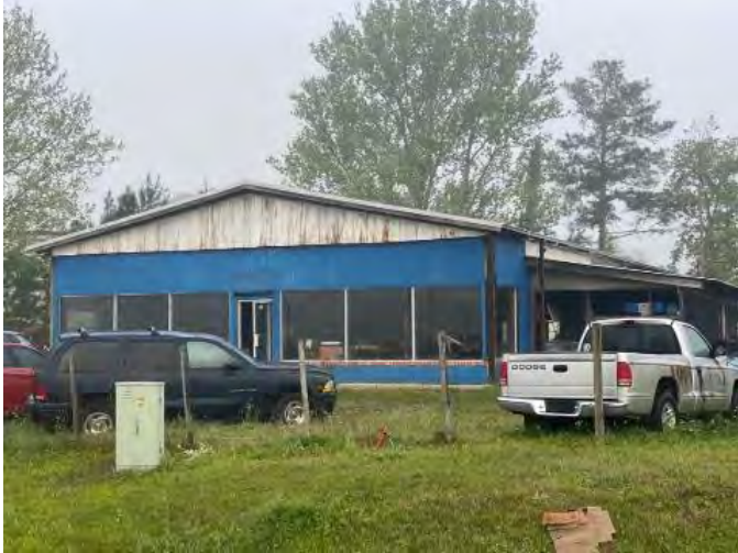
Figure 1216. Photograph of SJ07975 – 4 facing west.
