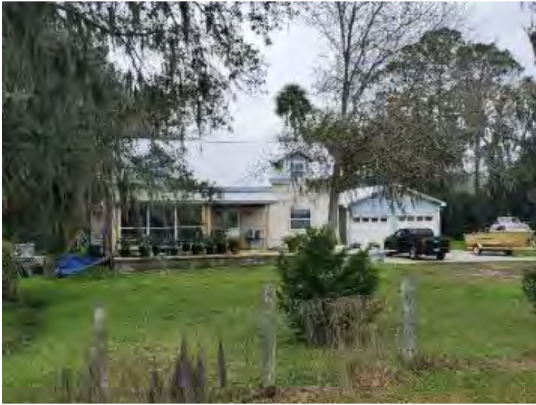
Figure 49. Photograph of SJ02594 – 2 facing west.
