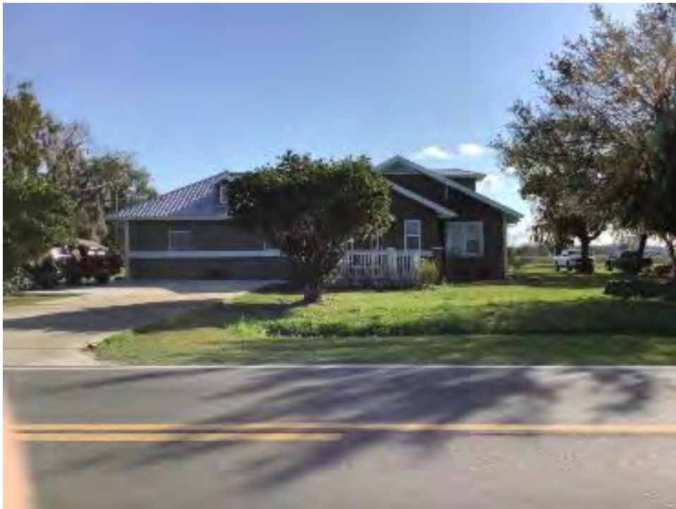
Figure 27. Photograph of SJ02584 – 2 facing east.
