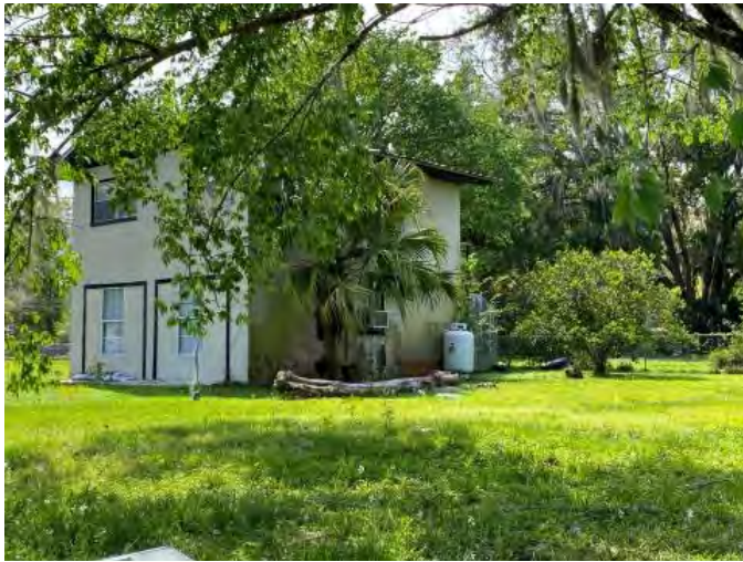
Figure 1141. Photograph of SJ07955 – 1 facing southwest.
