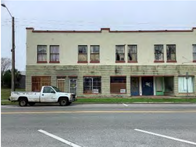
Figure 208. Photograph of SJ02704 – 2 facing west.
