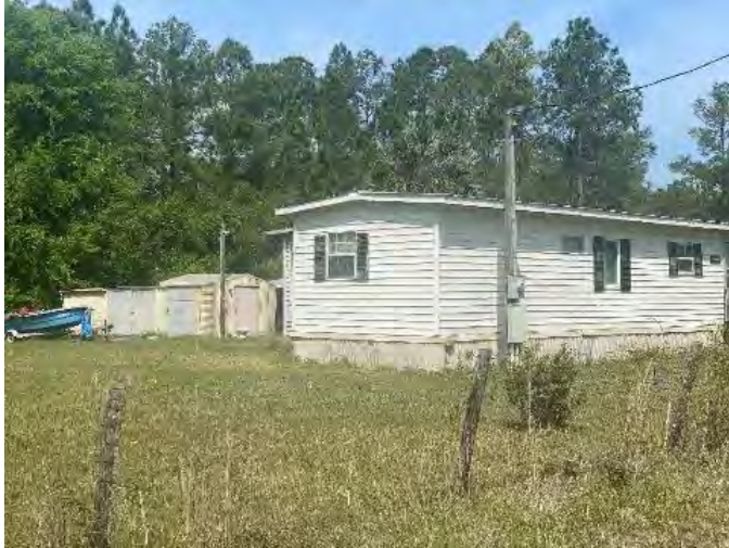
Figure 710. Photograph of SJ07827 – 3 facing south.
