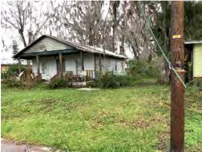
Figure 103. Photograph of SJ02661 – 3 facing west.
