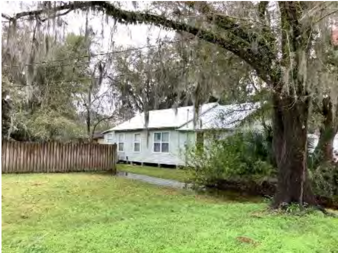
Figure 154. Photograph of SJ02681– 1 facing west.
