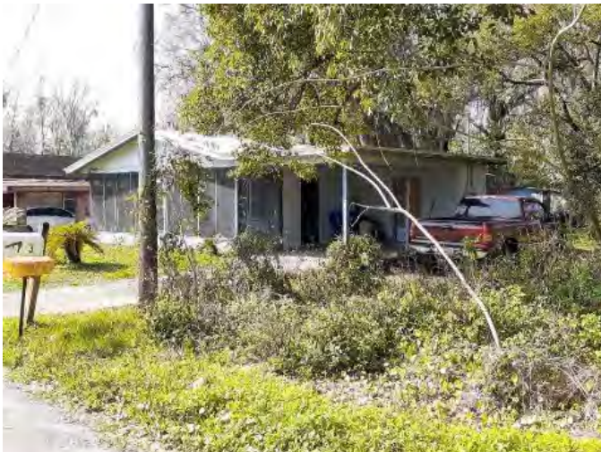
Figure 924. Photograph of SJ07892 – 3 facing northwest.
