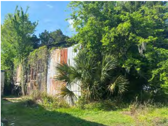
Figure 1041. Photograph of SJ07929 – 1 facing south.
