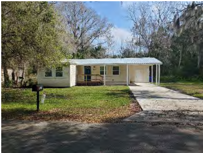
Figure 753. Photograph of SJ07839 – 1 facing east.
