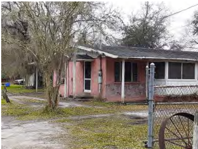
Figure 1005. Photograph of SJ07917 – 2 facing southwest.
