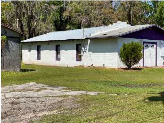
Figure 1155. Photograph of SJ07959 – 1 facing northwest.
