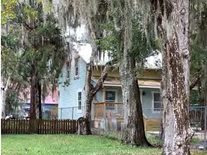
Figure 446. Photograph of SJ07752 – 2 facing southwest.
