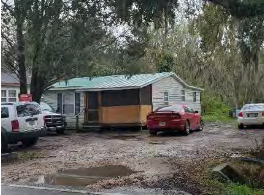
Figure 584. Photograph of SJ07792– 1 facing south.
