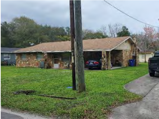
Figure 358. Photograph of SJ07726 – 2 facing northwest.
