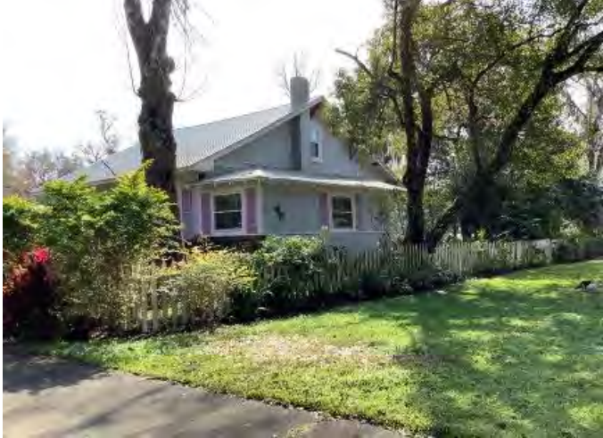
Figure 525. Photograph of SJ07774 – 3 facing east.
