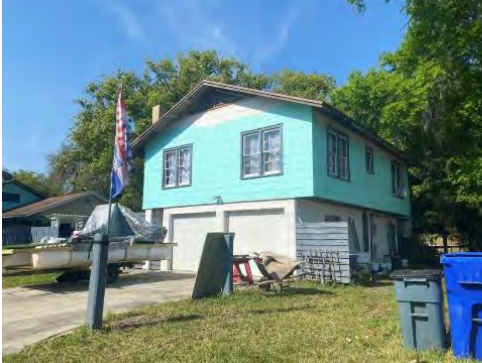
Figure 1058. Photograph of SJ07933 – 3 facing southwest.
