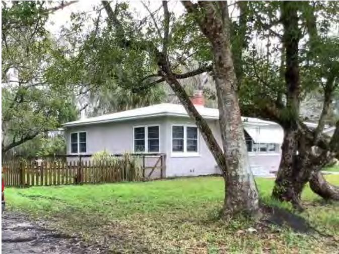
Figure 392. Photograph of SJ07736 – 2 facing east.
