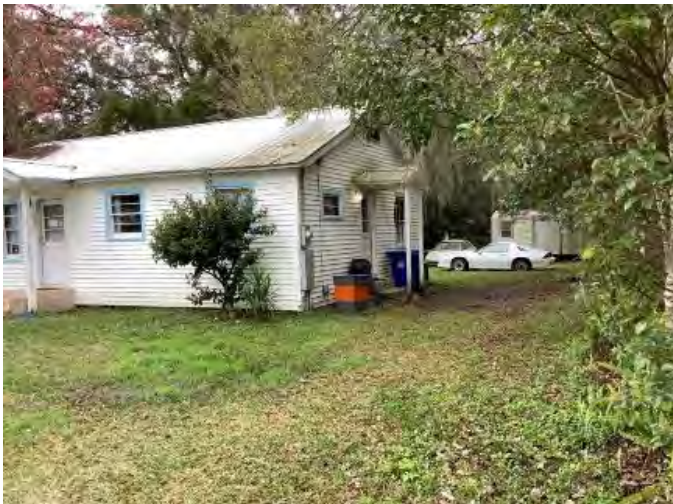
Figure 660. Photograph of SJ07812 – 3 facing east.
