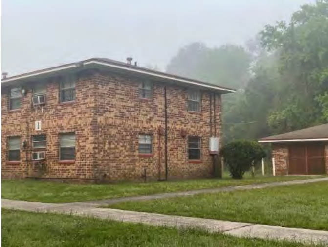
Figure 1188. Photograph of SJ07968 – 1 facing southwest.
