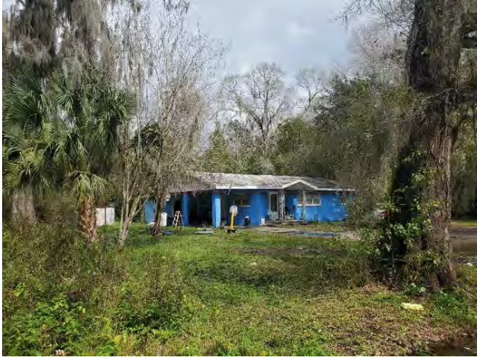
Figure 692. Photograph of SJ07821 – 1 facing northwest.
