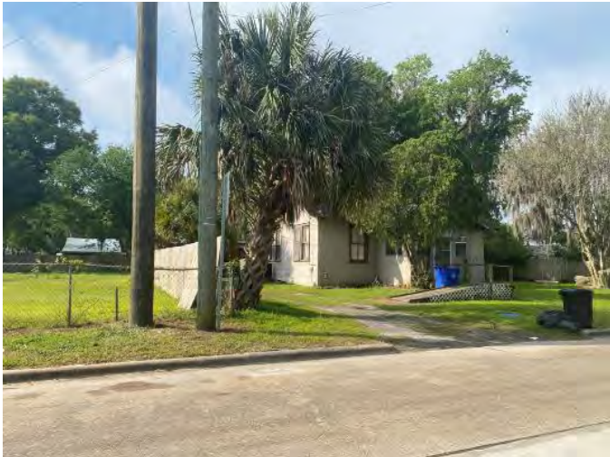
Figure 1092. Photograph of SJ07942 – 3 facing south.
