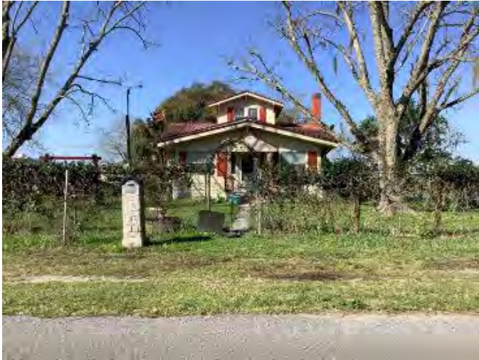
Figure 239. Photograph of SJ03114 – 2 facing west.
