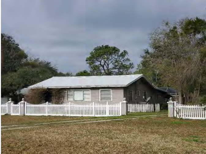
Figure 785. Photograph of SJ07849 – 1 facing southwest.
