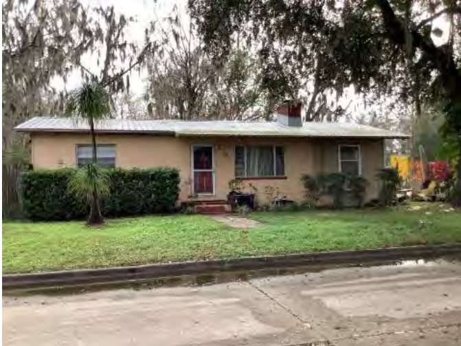
Figure 488. Photograph of SJ07765 – 1 facing east.
