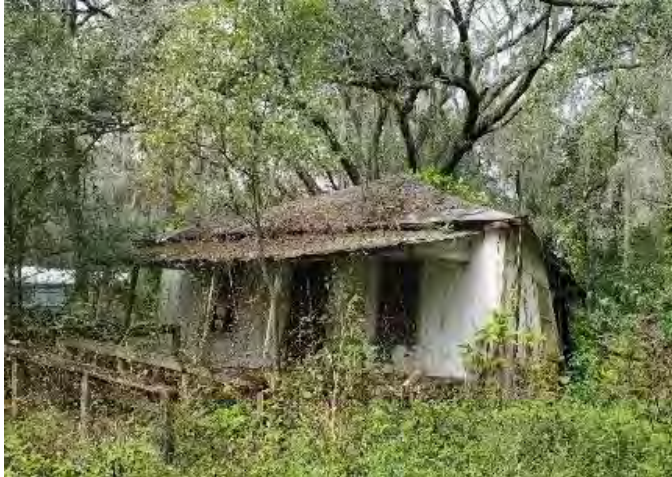
Figure 668. Photograph of SJ07814 – 3 facing west.
