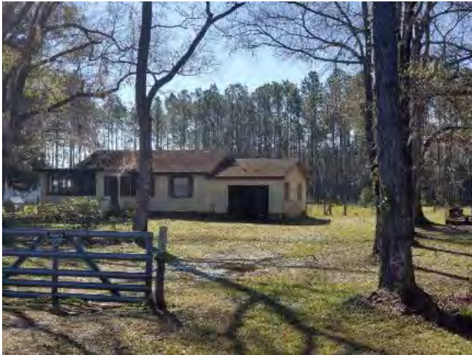
Figure 650. Photograph of SJ0809 – 3 facing south.
