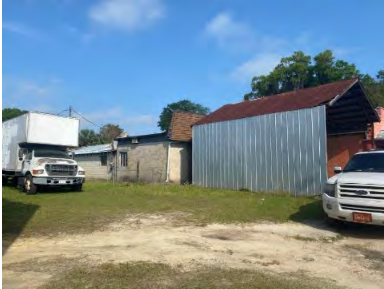
Figure 1125. Photograph of SJ07951 – 2 facing northwest.
