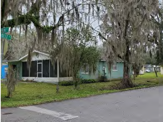
Figure 836. Photograph of SJ07863 – 3 facing southwest.
