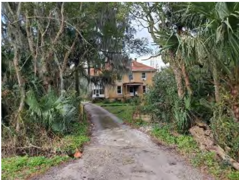
Figure 40. Photograph of SJ02590 – 1 facing west.
