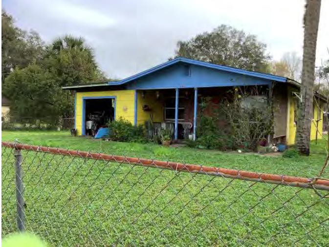
Figure 716. Photograph of SJ07829 – 1 facing east.
