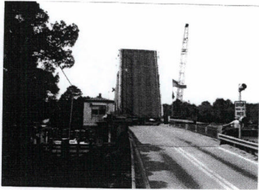
Figure 26: Palm Valley Bridge, 1937
