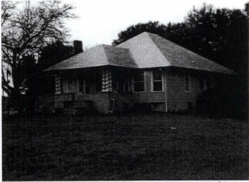
Figure 15: Sears, Roebuck & Company's "Avondale" at Elkton, c. 1912
