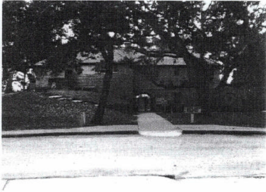
Figure 41: Rustic Style, Visitor's Center, 1937, Matanzas National Monument
