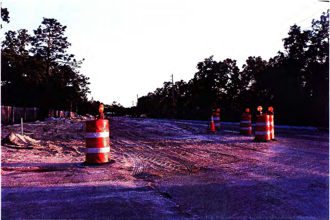
Road construction south of Switzerland widening State Road 13 to four lanes
