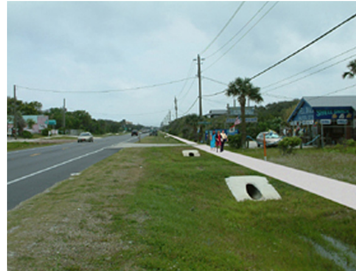
After sidewalk installation
