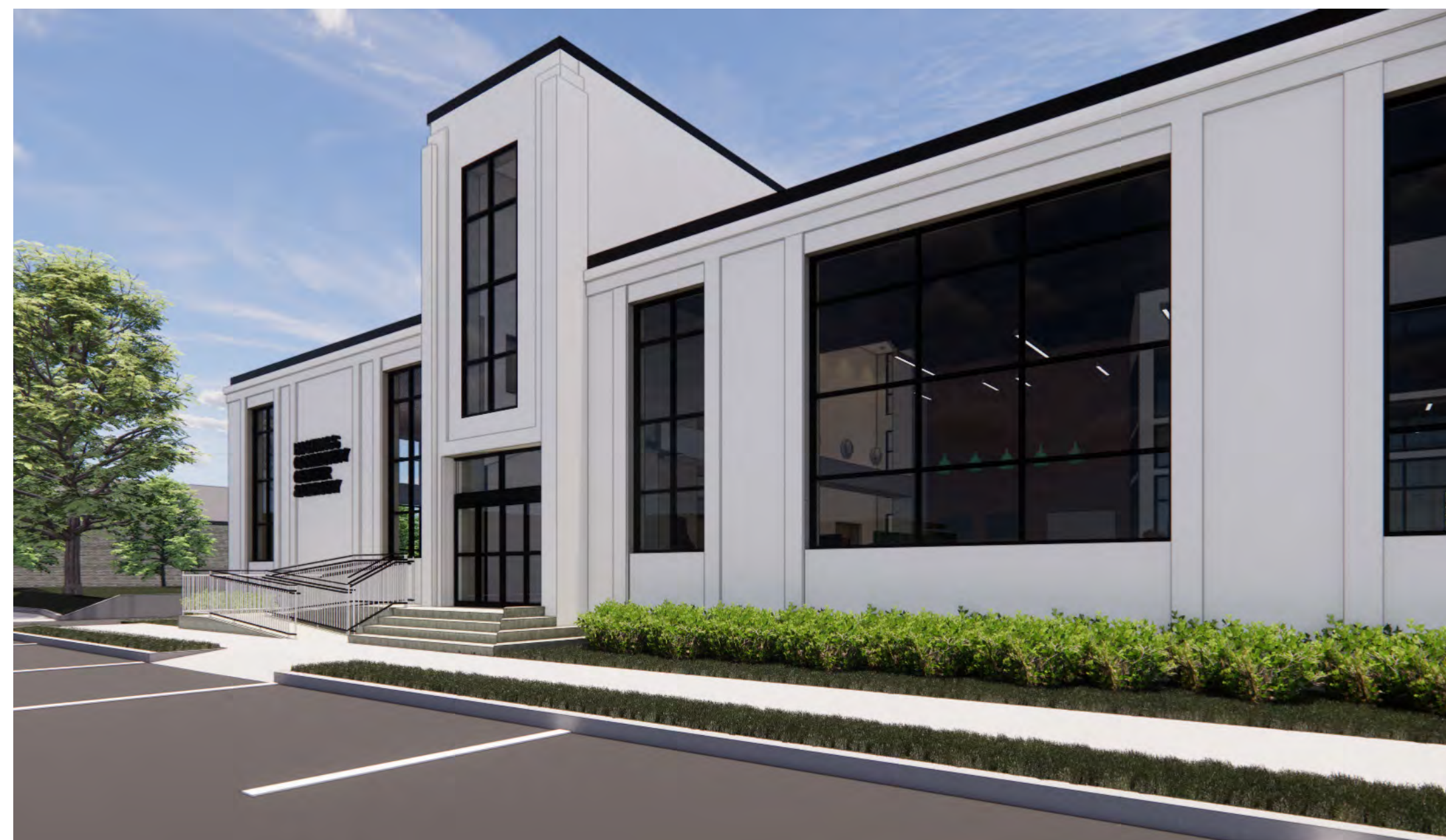
EAST ENTRY MAIN STREET SIDE/APPROACHING THE BUILDING
