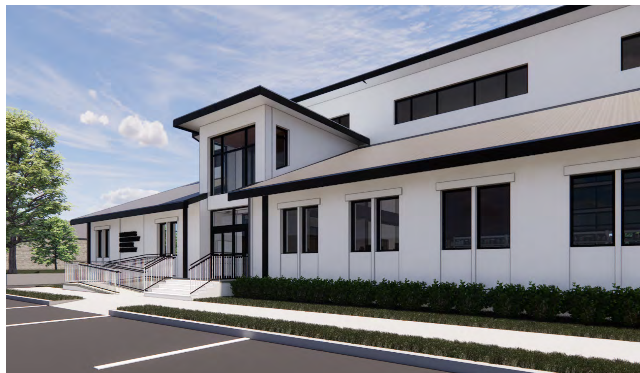
EAST ENTRY MAIN STREET SIDE/APPROACHING THE BUILDING
