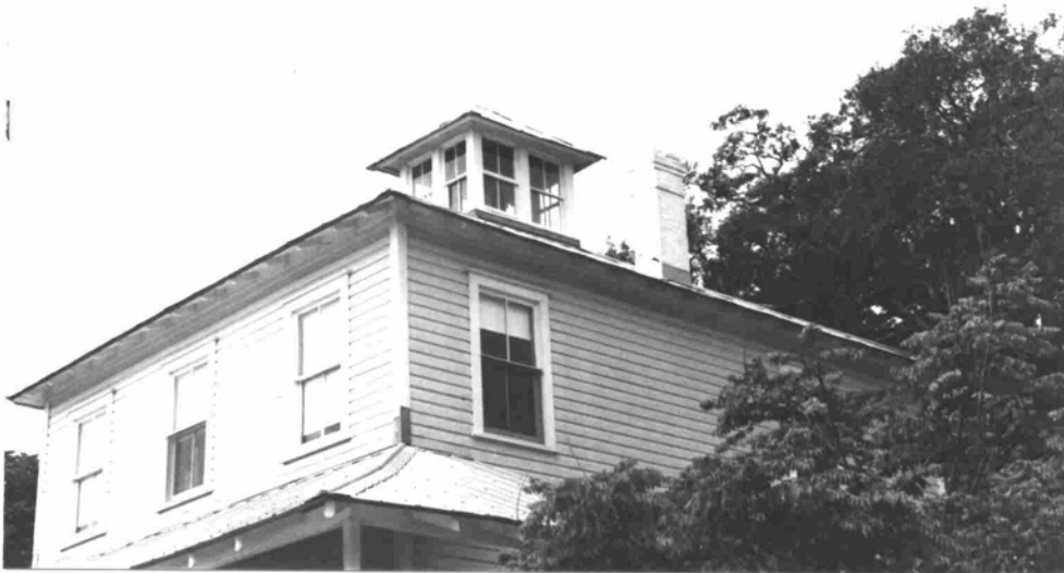
Photo #6 Details of Facade - N.E. Corner
