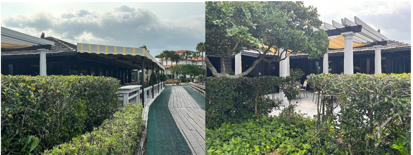
Figures 3A-B: Existing Conditions —Staff Photographs of Existing Conditions, taken April 11, 2024.
