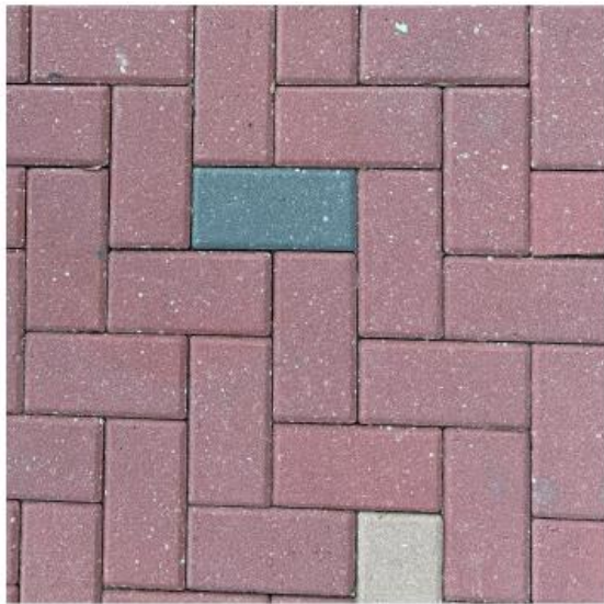
4" X 8" CONCRETE PAVER HERRINGBONE PATTERN COLOR: HERITAGE (PRIMARY COLOR) 2%-5% RANDOM MIX OF CHARCOAL AND TAN BY TREMOR (OR SIMILAR) MATCH EXISTING PAVER PATTERNS AND MIX USED FOR OTHER PATIO AREAS
