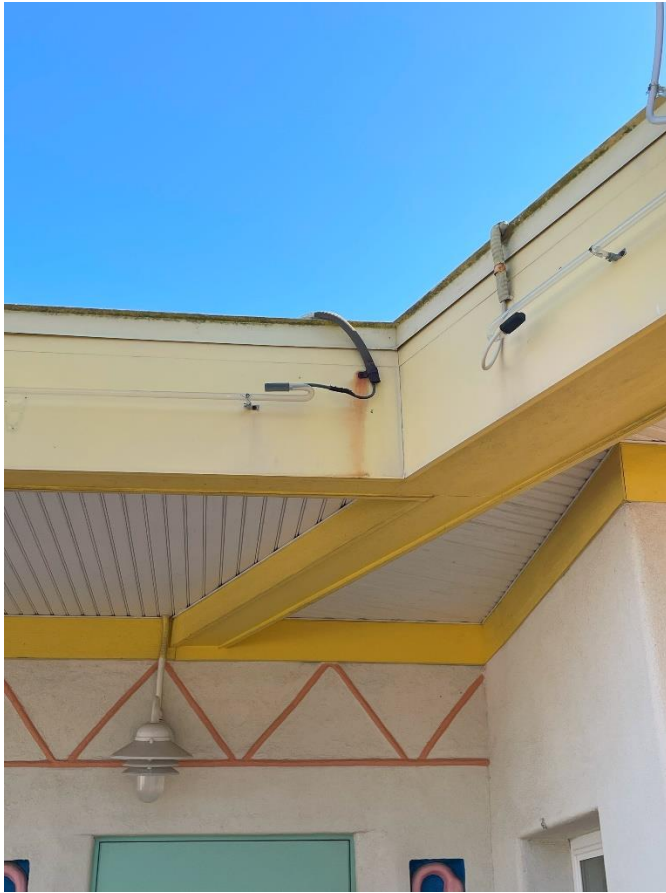
Newer neon lighting installed on the building fascia. Note the power is improperly terminated and the cables simply laid on the roof or in the gutters.
