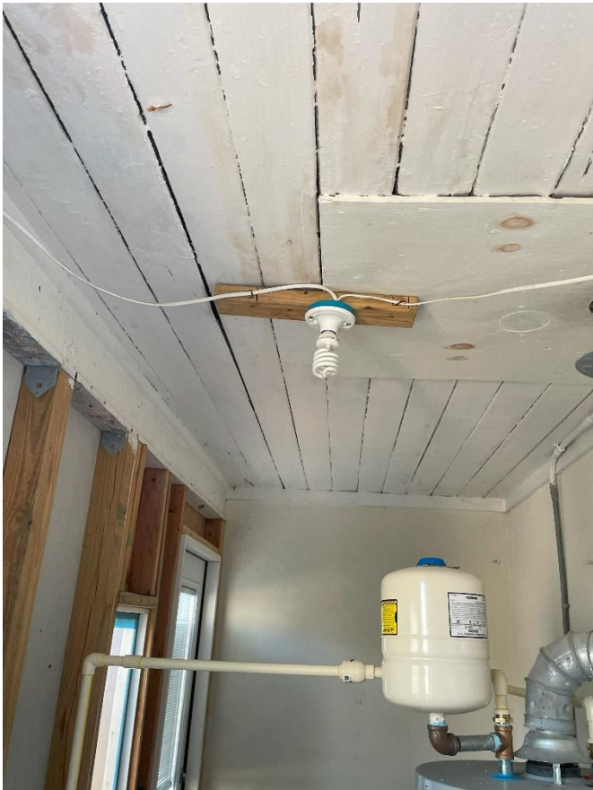
Utility room with improper electrical wiring. This occurs frequently around the building.
