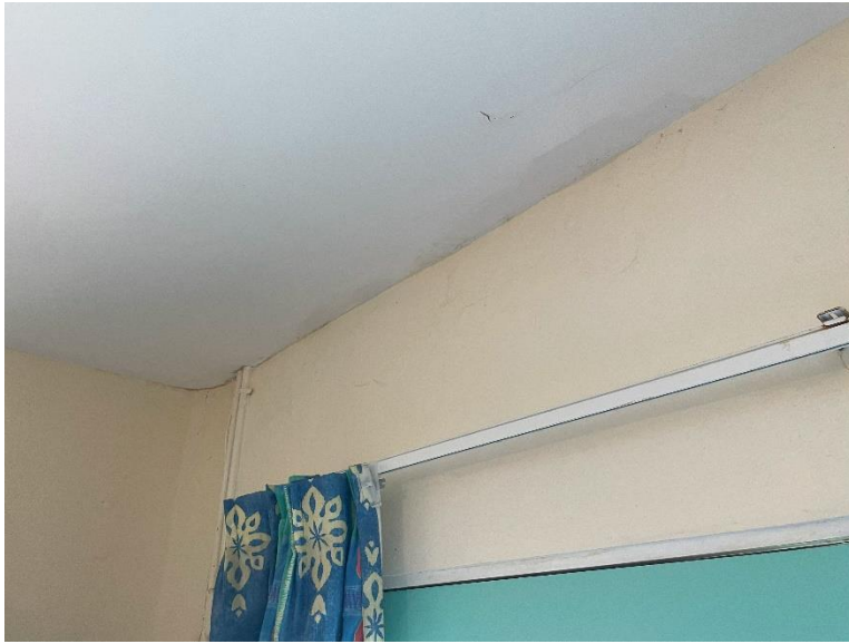
Evidence of roof leakage in another guest room.
