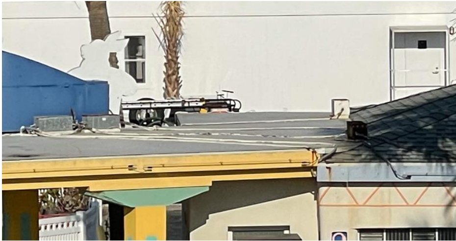
The roof is home to multiple transformers and switches for the neon lighting that was added by the TV show. Wiring is improperly laid on the roof.
