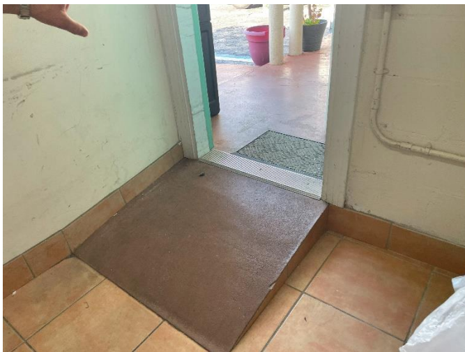
The finished floor of portions of the hotel are below the exterior grade.
