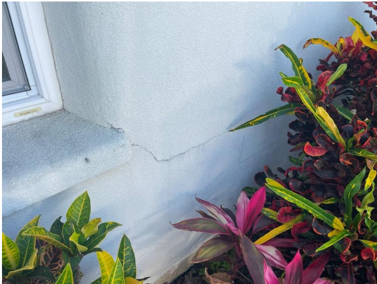
The building has been wrapped in EFIS (a newer material) and yet CMU cracking is still visible. Foundations have settled to cause the cracking seen in the walls.
