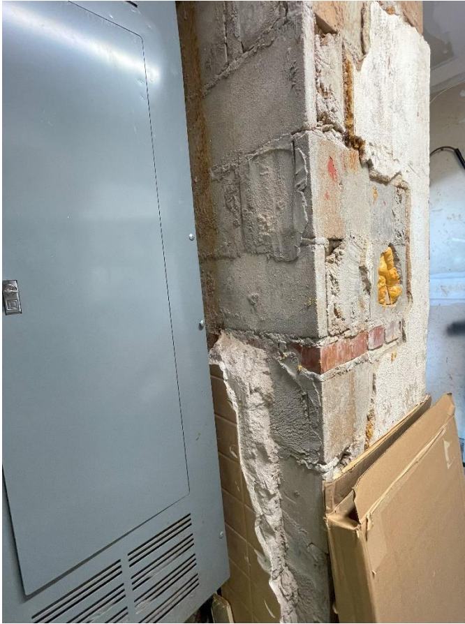
Poor original construction. Note: The chimney construction a mix of CMU and brick with terrible workmanship.
