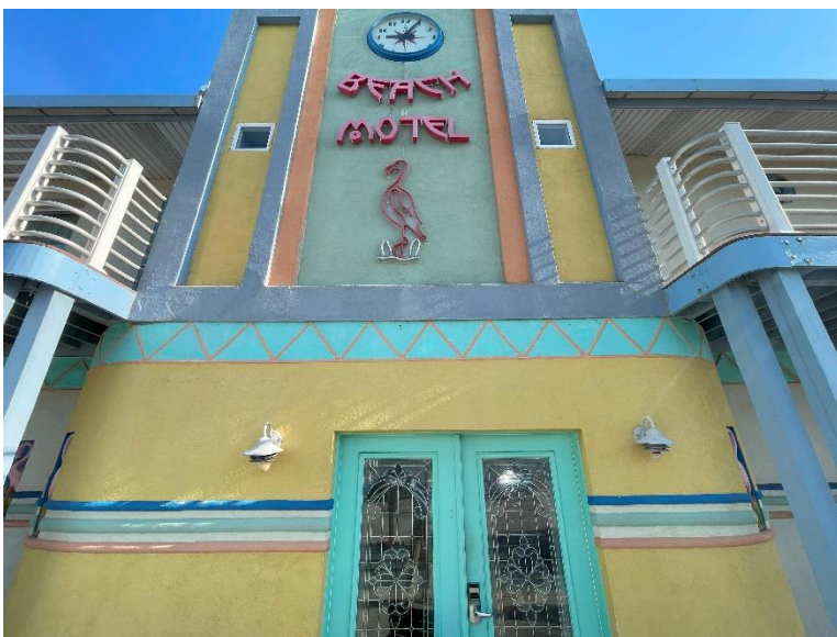
This is the most successful Art Deco example on the building. This is an addition from 20+/- years ago. The wall flashing is not installed and the wall leaks into the first-floor room below.
