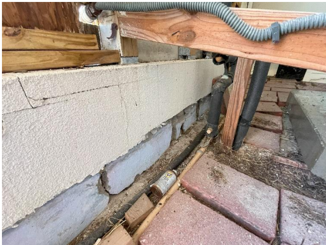
Extremely poor construction conditions. This wall condition is concerning. Observed open gaps in the CMU wall system, no concrete slab (pavers), standard wood verse pressure treated at the masonry.
