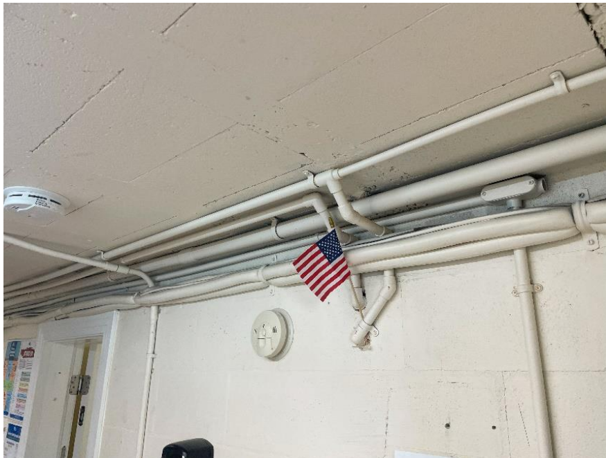
A mix of electrical conduit and water piping run in a hap-hazard way.
