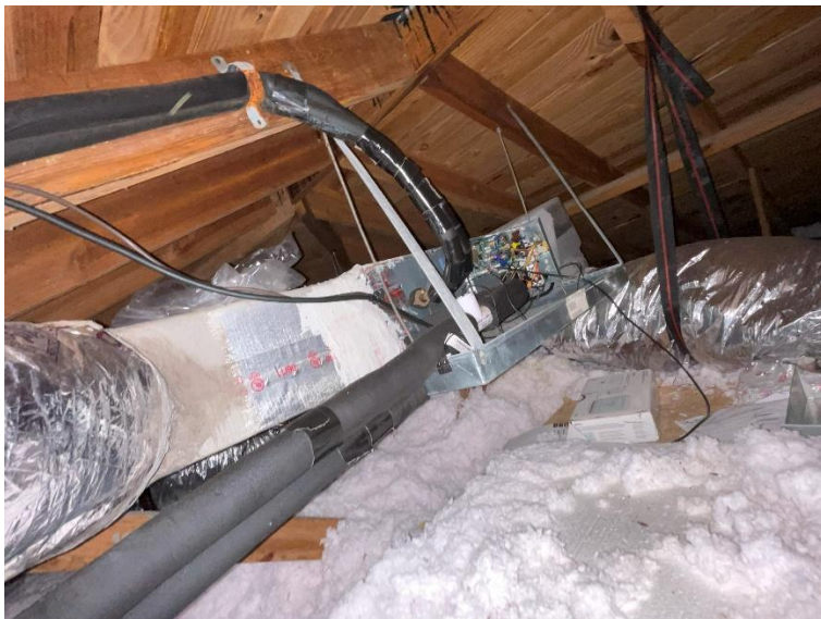
Poor original construction conditions. The air conditioning has been retrofitted post original building and located in an unconditioned attic not meeting code. Note that no rafters or beams have any type of hurricane clip or metal strapping.
