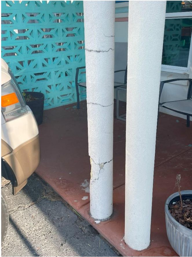
No curb line to restrict vehicles from colliding with structural columns supporting the building. Note column has been hit by a vehicle.
