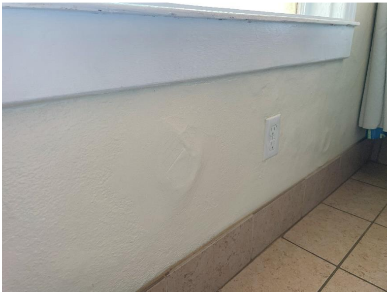
Evidence of water leakage in the wall and window system is prevalent in most guest rooms.
