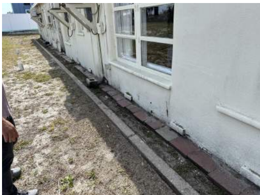
Photo Showing Grade at Rear Wall
