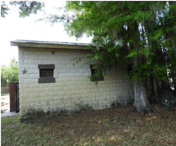
Rear of Structure
