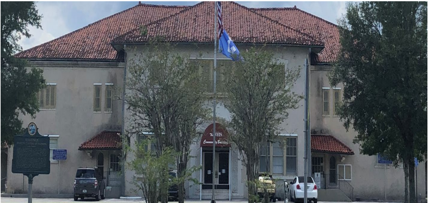
Former Hastings High School Building
