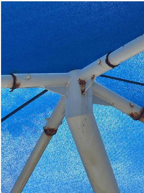
Shade Structure Deterioration:
