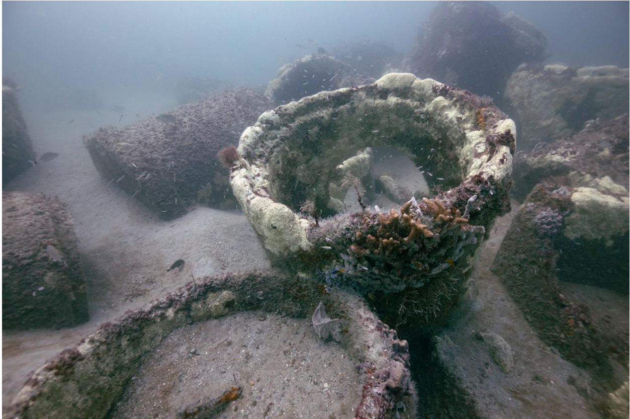
Figure 4 Underwater View of Encrusted Concrete Culverts During the Dive Investigation
