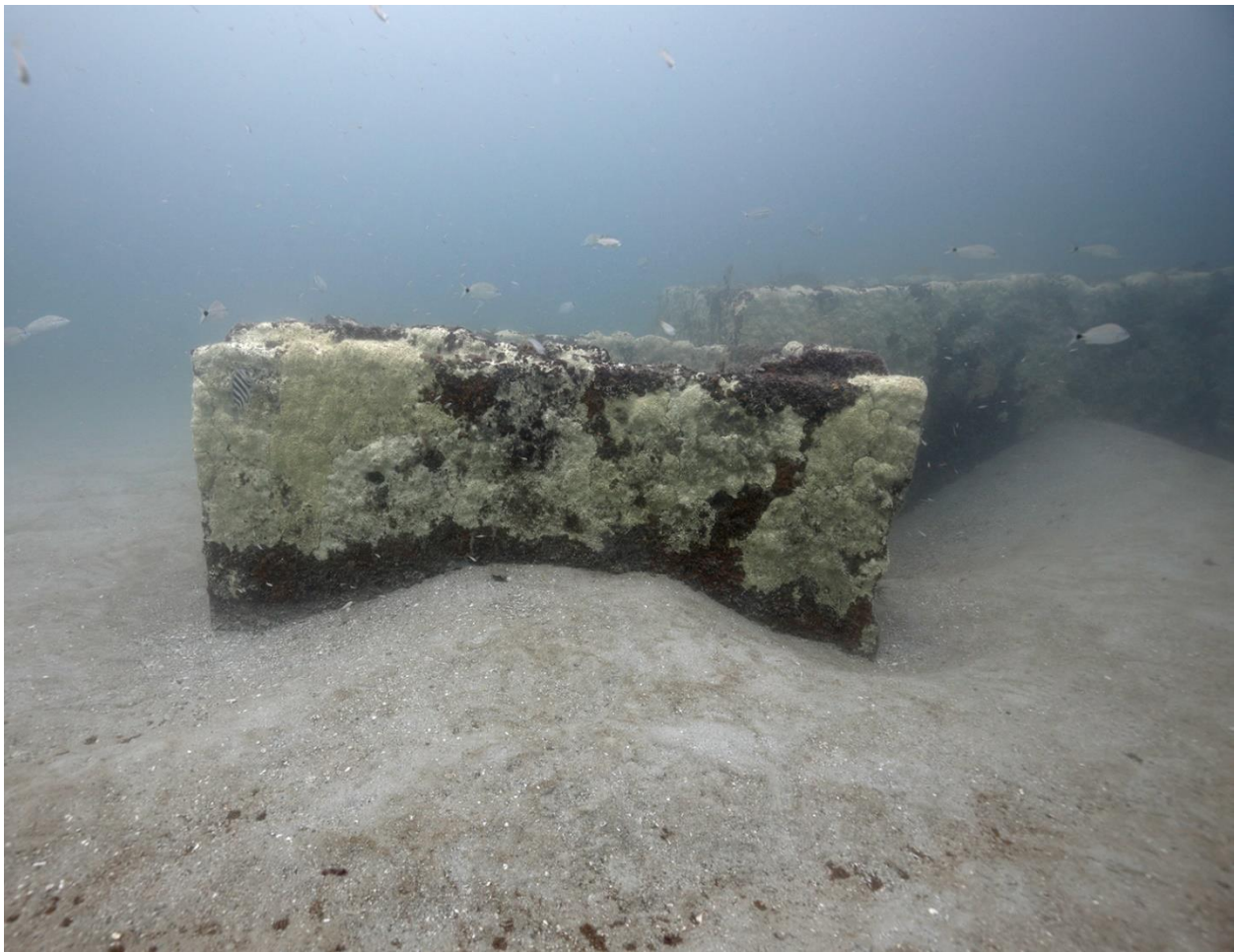
Figure 6: Sand Excavations Caused by Marine Life
