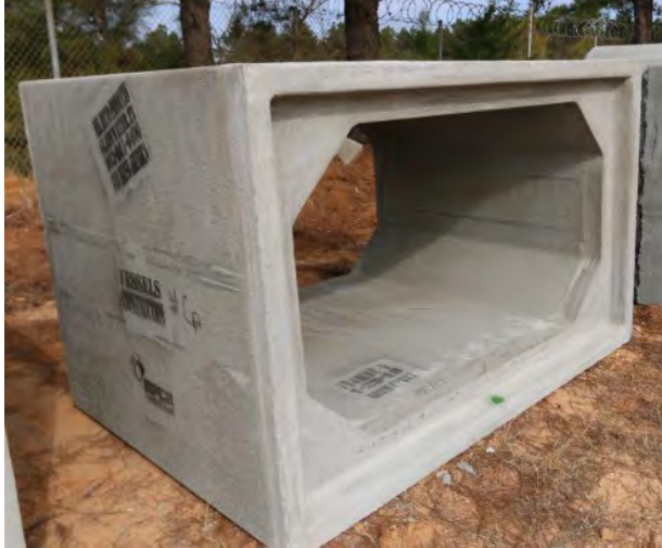
Figure 106 - Typical Concrete Culverts on Moody
