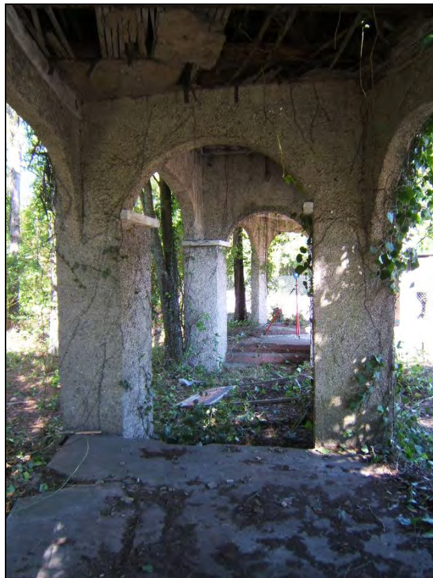
View of Arch from inside Looking Northwest
