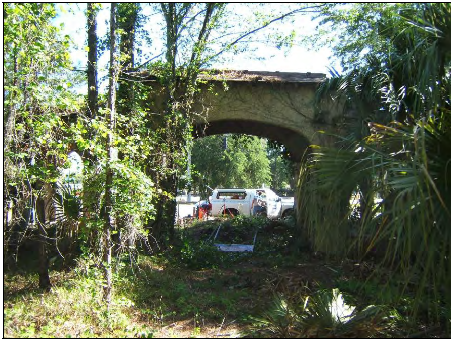
View of Arch Looking Northeast from Campus
