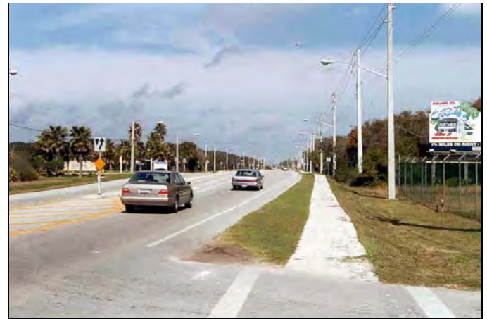
Overhead utilities along SR A1A
