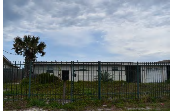
Photograph 101. SJ05450, 2877 South Ponte Vedra Boulevard.
