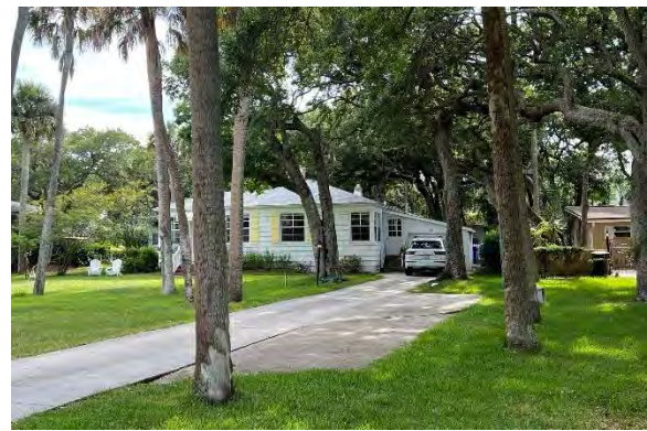
Photograph 22. SJ03770, 54 San Juan Drive.
