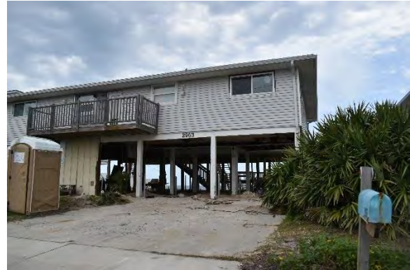
Photograph 173. SJ08113, 2963 South Ponte Vedra Boulevard.
