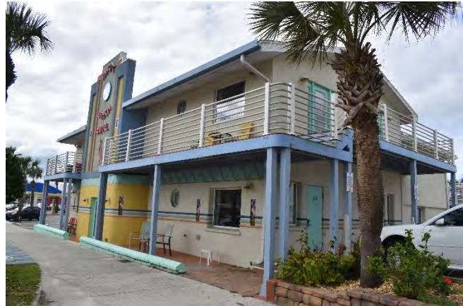
Photograph 8. Streamline Moderne Building, 50 Vilano Road.
