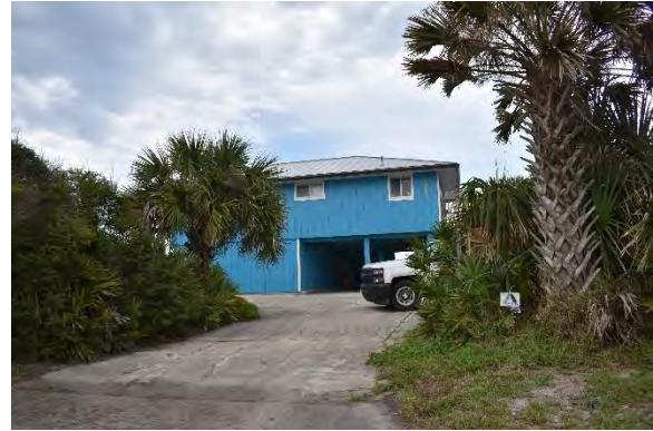
Photograph 171. SJ08111, 2967 South Ponte Vedra Boulevard.
