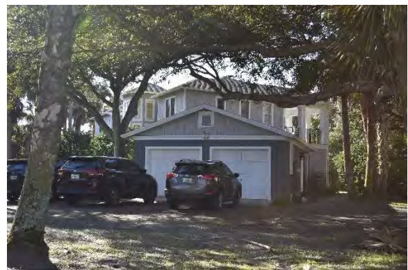
Photograph 25. SJ03774, 51 San Juan Drive.
