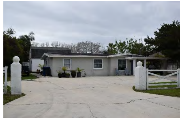
Photograph 125. SJ08065, 109 Morgan Avenue.
