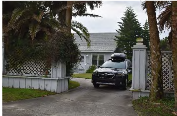
Photograph 100. SJ05448, 11 Oak Avenue / 31-A Oak Avenue.
