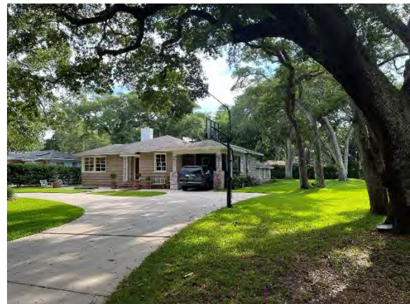
Photograph 23. SJ03771, 58 San Juan Drive.
