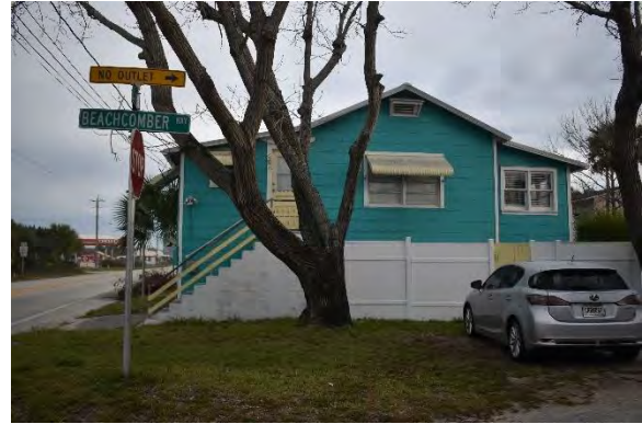
Photograph 77. SJ03914, 50 Beachcomber Way.
