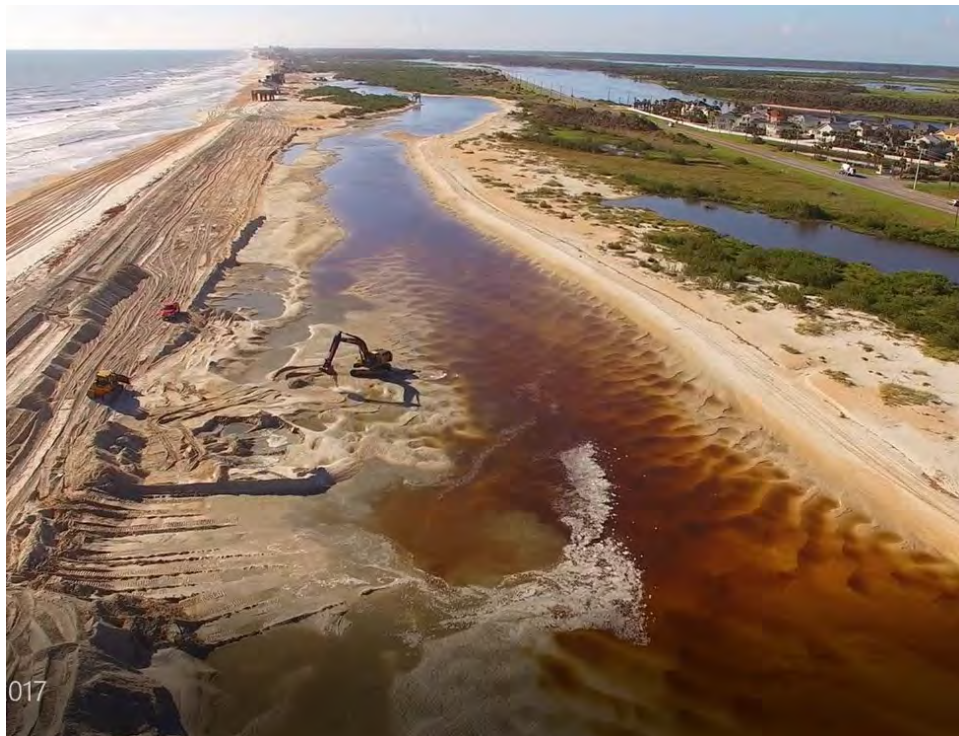
Figure 2.9 North End - Post-Hurricane Irma Re-construction (Taylor Engineering, 2018)
