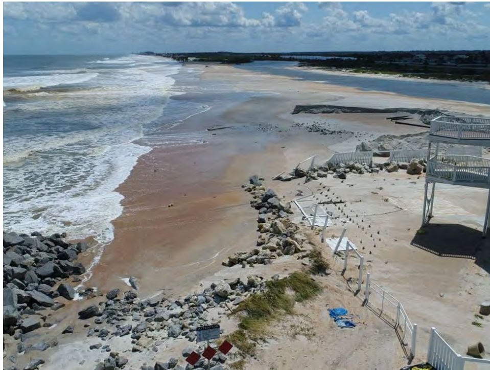
Figure 2.8 North End - September 2017 Post-Hurricane Irma (Taylor Engineering, 2018)
