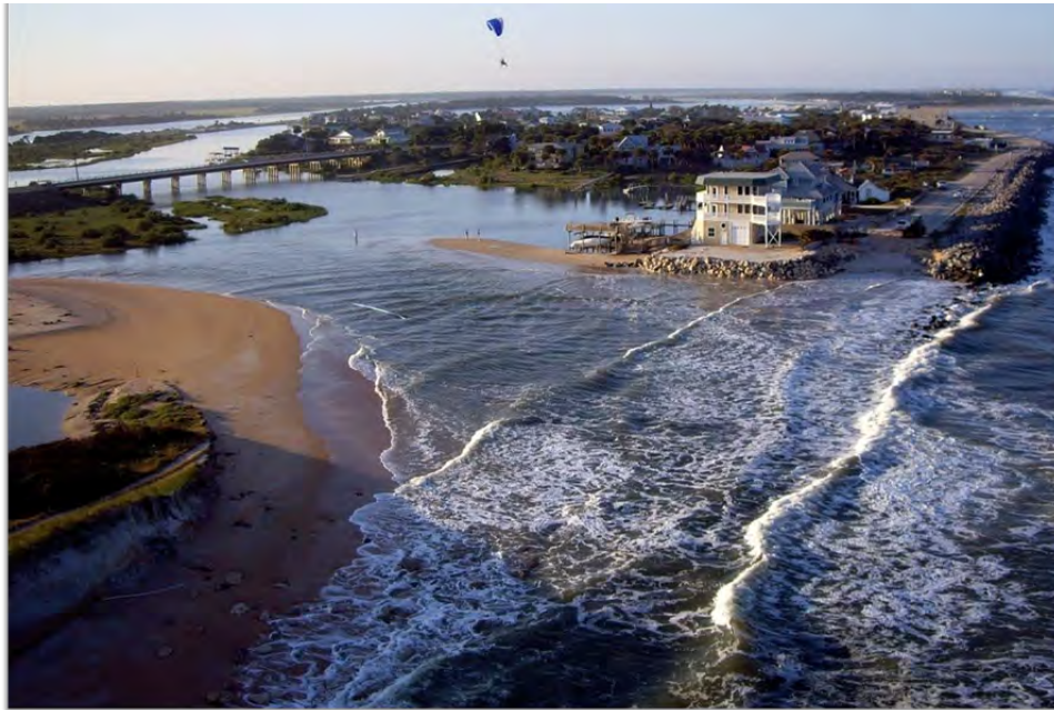
Figure 2.4 North End - 2008 Tropical Storm Fay Breach (Taylor Engineering, 2018)
