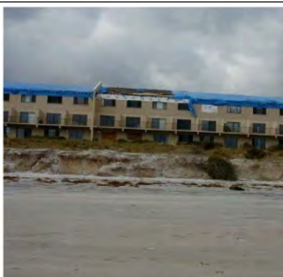
Photo 1 Anastasia Island Erosion at R-193
