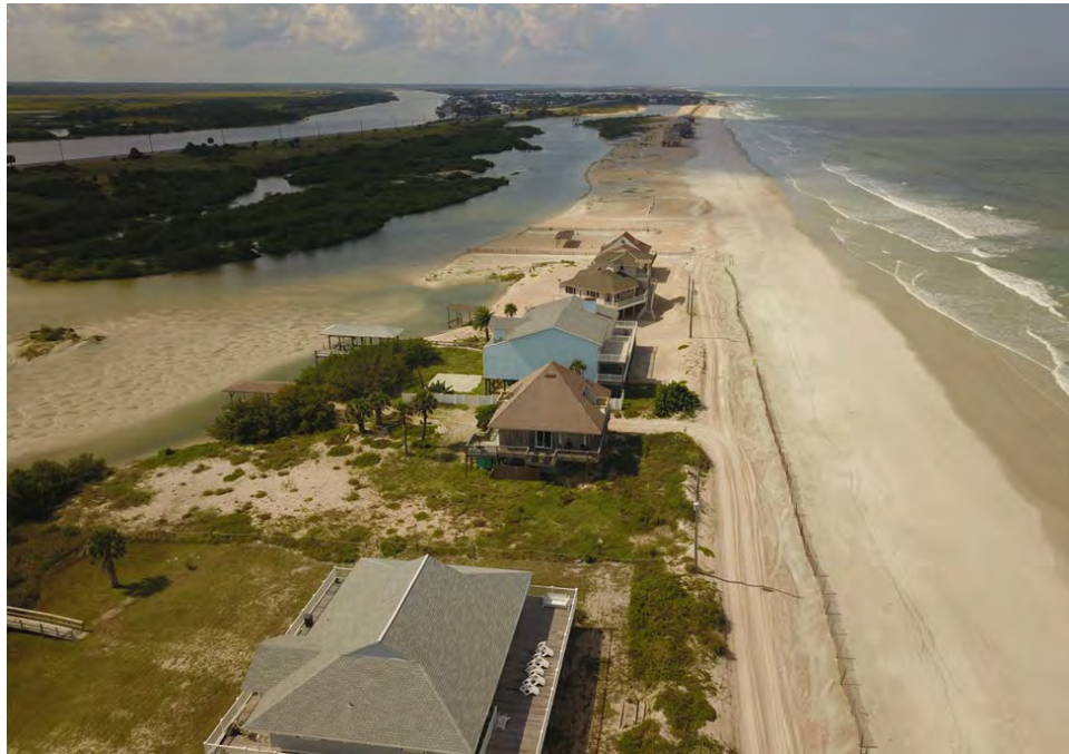
Figure 2.16 South End - August 2019 Pre-Hurricane Dorian (source: St. Johns County)
