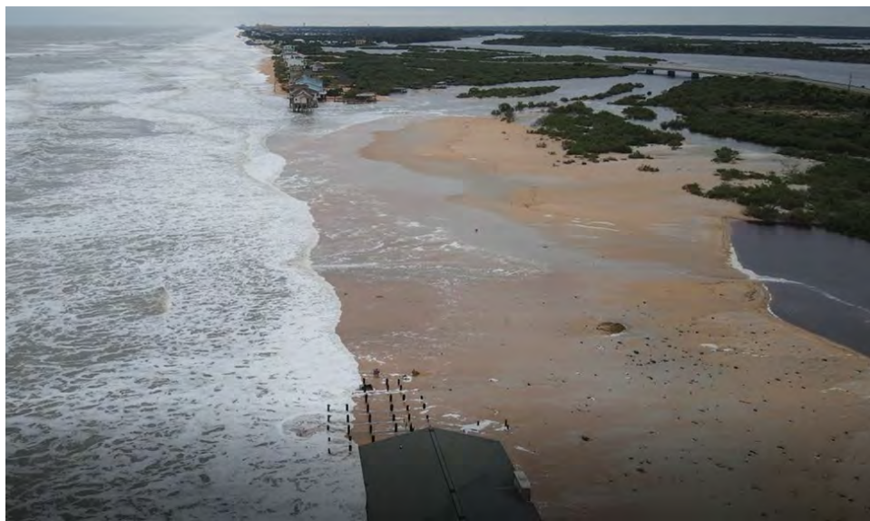
Figure 2.15 South End – September 2017 Post-Hurricane Irma Breach (source: St. Johns County)
