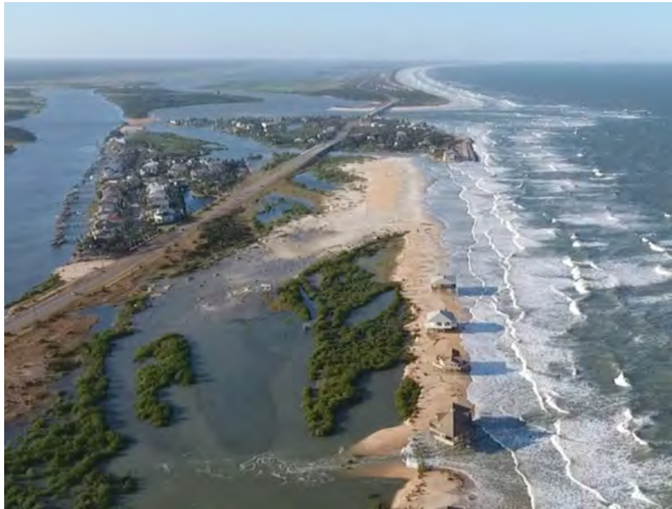
Figure 2.6 North End - October 2016 Post-Hurricane Matthew (Taylor Engineering, 2018)
