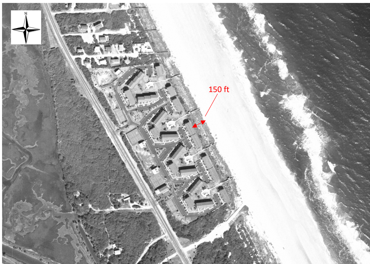
Figure 2.3 Aerial Acquired Feb 1993 ( https://fdotewp1.dot.state.fl.us/aerialphotolookupsystem )
